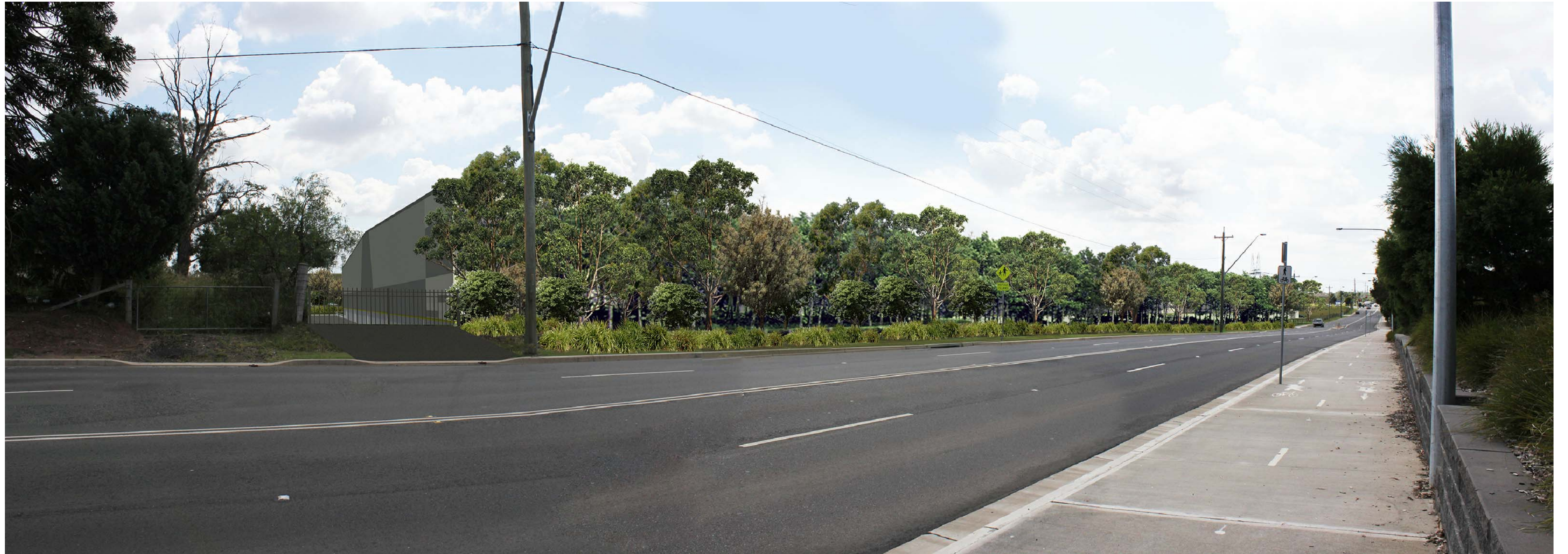
VIEW FROM SOUTH WEST GROUND LEVEL VIEW ALONG KURRAJONG ROAD LOOKING TOWARDS EAST DIRECTION
