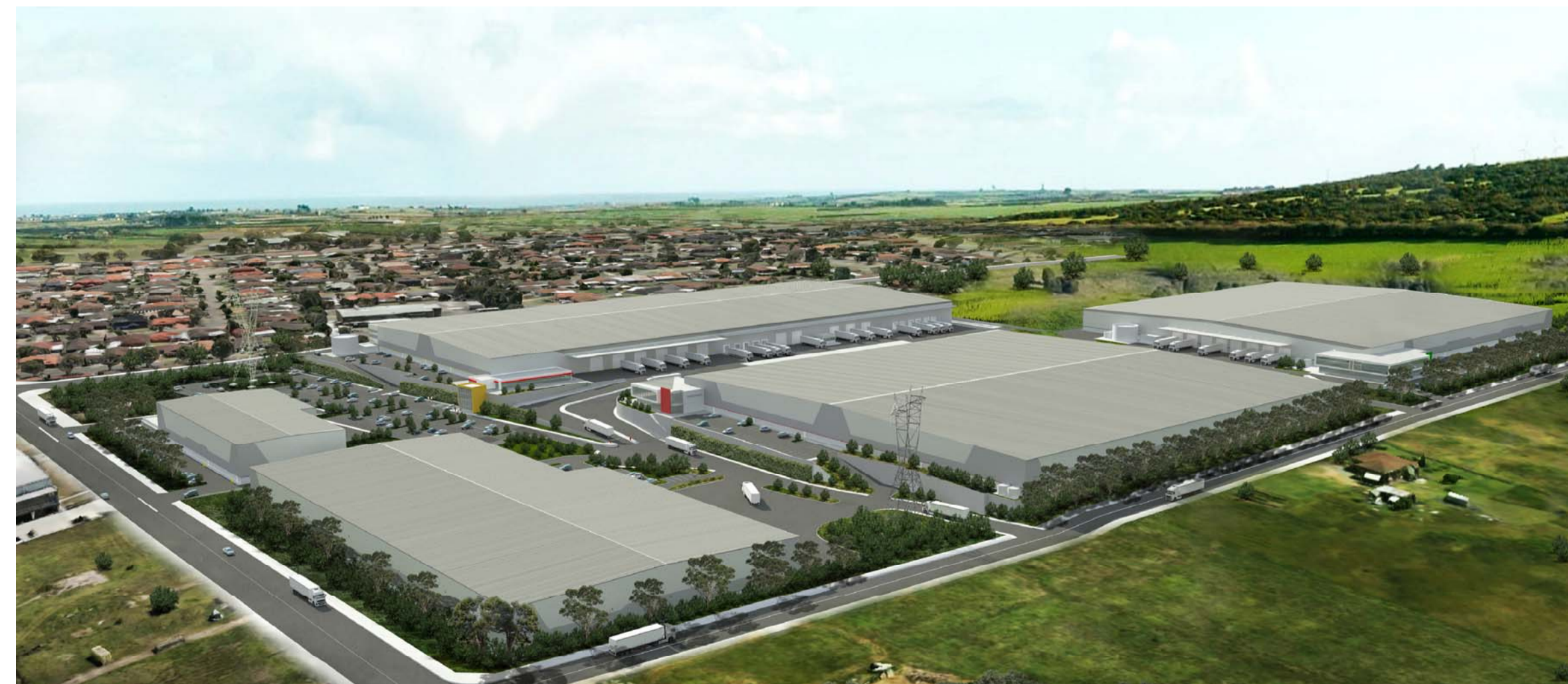
VIEW FROM NORTH EAST
