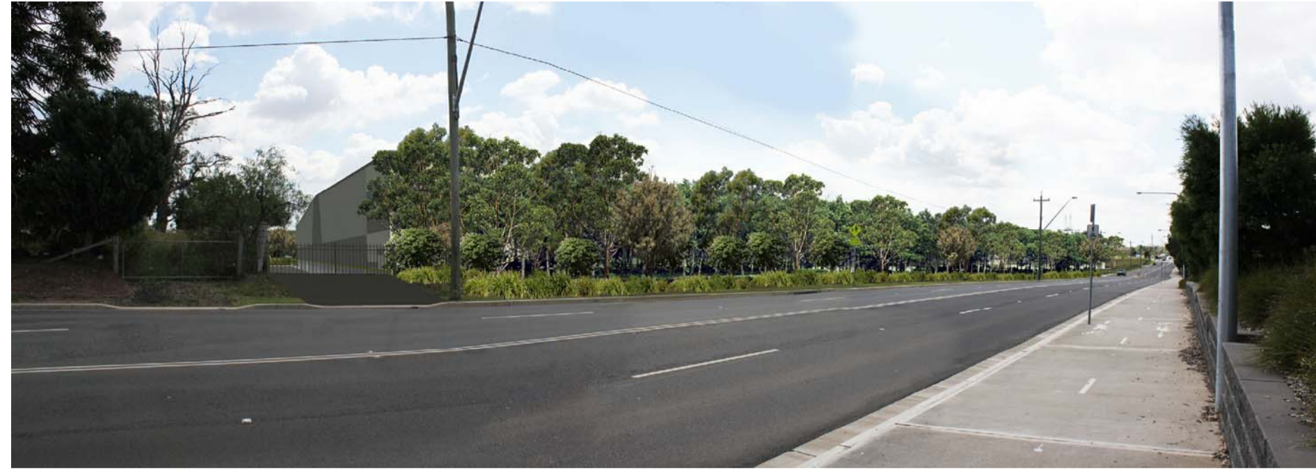
VIEW FROM SOUTH WEST (street level view of warehouse 5 along Kurradjong Road)
