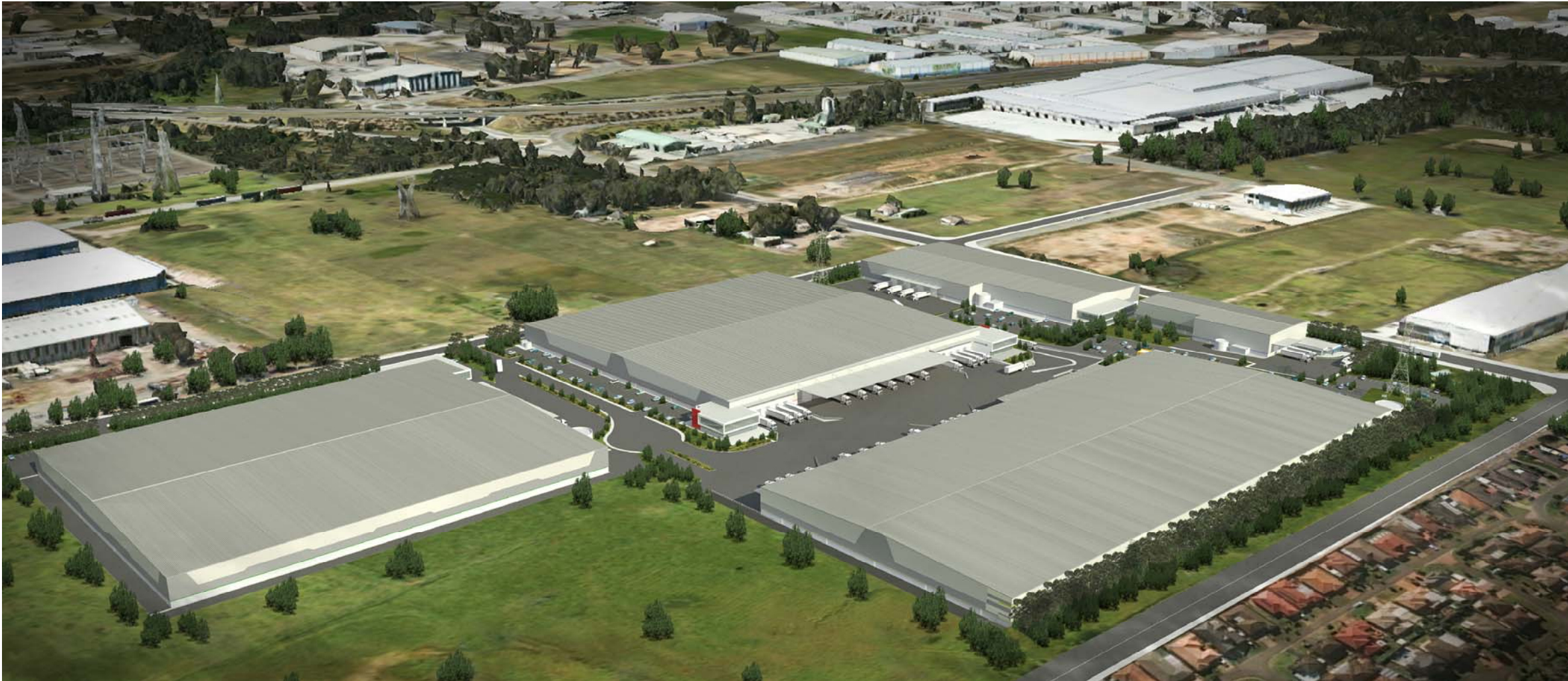
VIEW FROM SOUTH WEST
