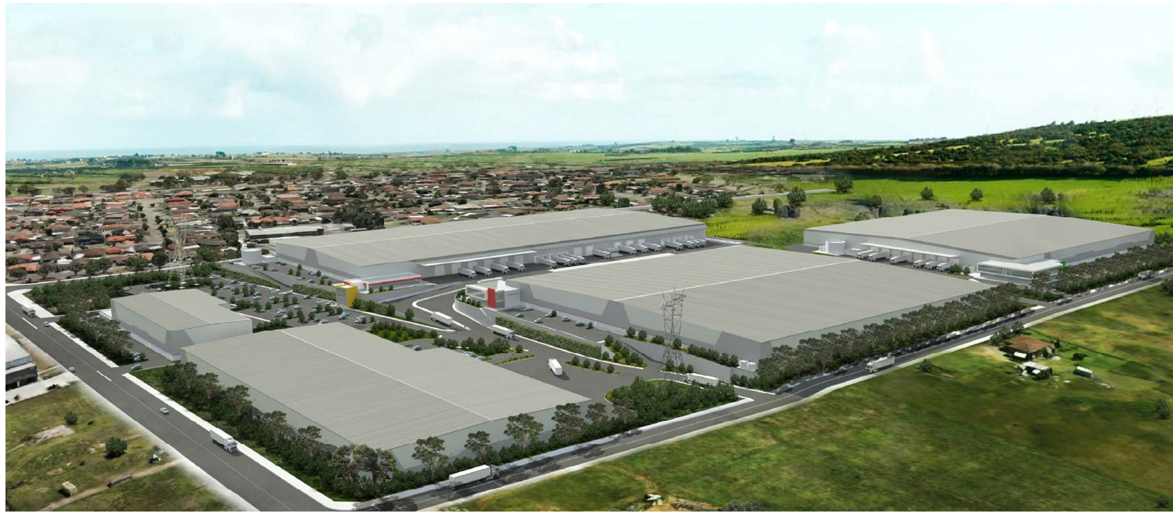
VIEW FROM NORTH EAST
