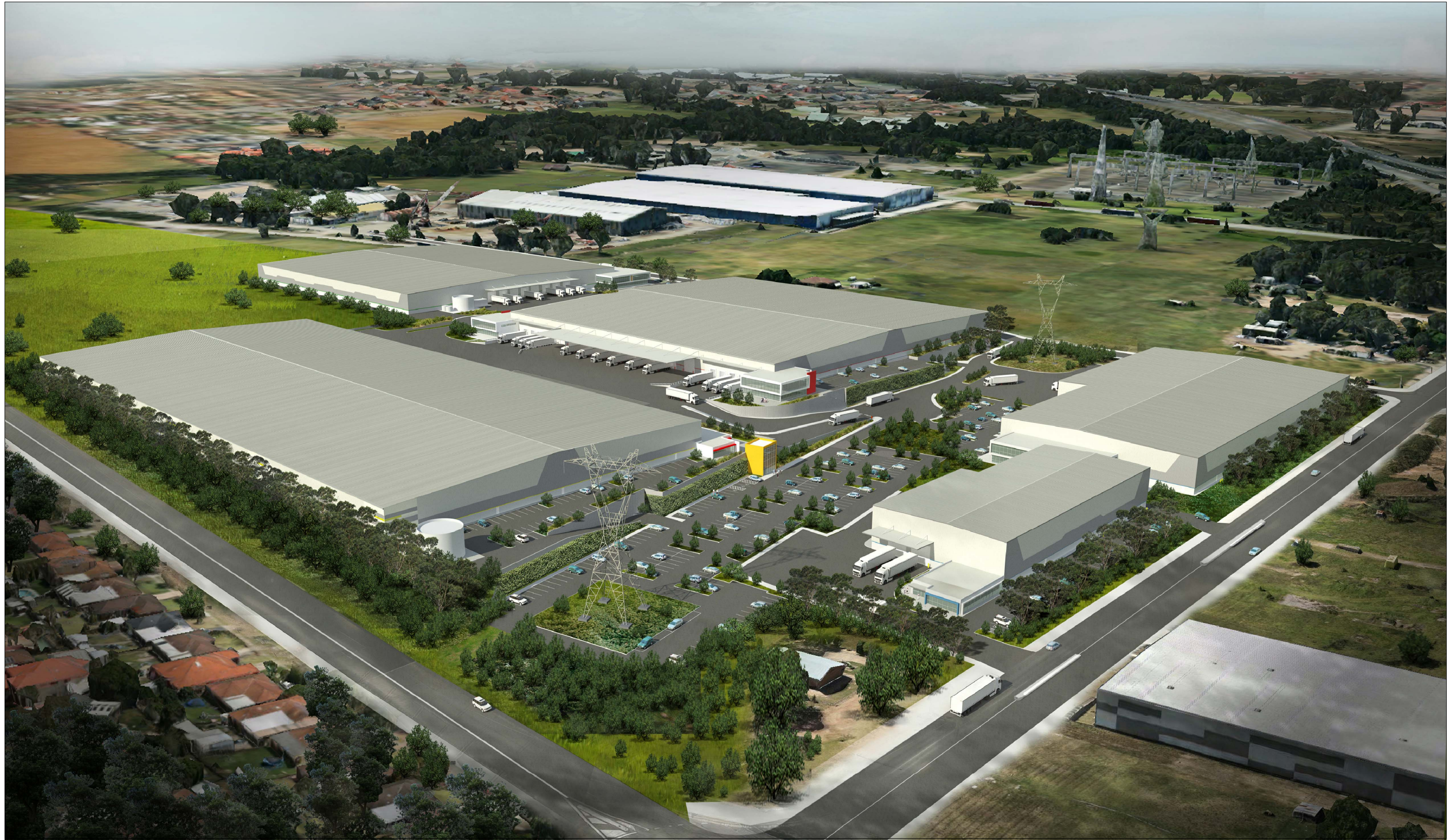
AERIAL VIEW FROM SOUTH EAST
