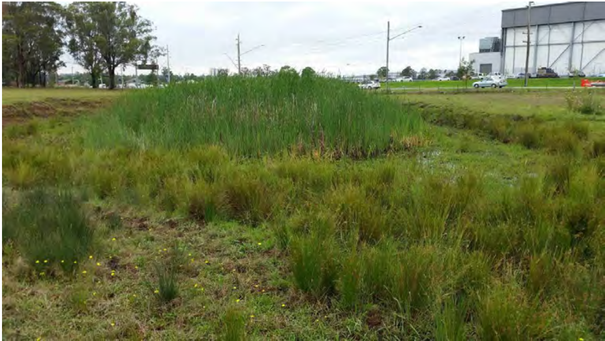
Photo 6 – The dam and fringing vegetation
