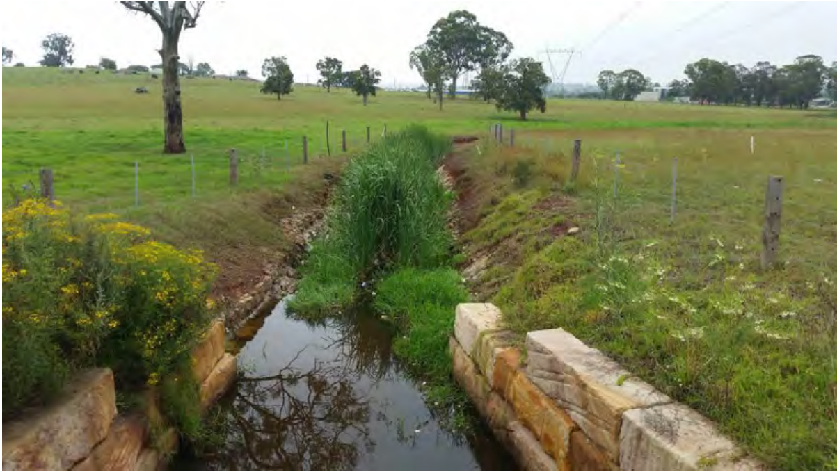
Photo 8 – Constructed drainage off Kurrajong Road adjacent to the electrical easement
