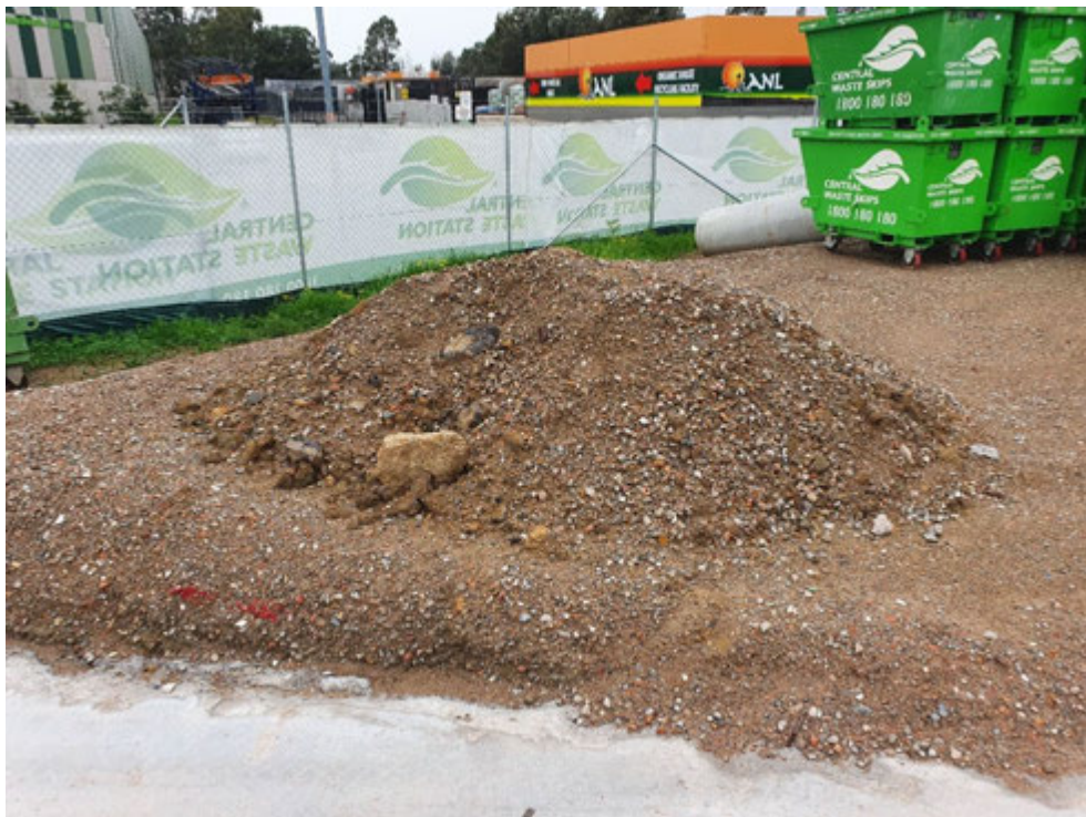
Photograph 6 – Excess recovered aggregate stored around perimeter of Site.
