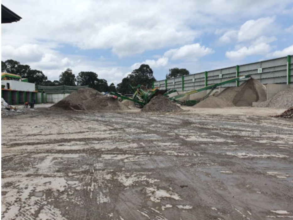
Photograph 5 – (8 Styles St) Recycled concrete and brick aggregate stockpiles. Material is periodically wet down to reduce dust generation potential.
