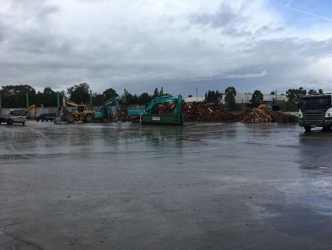
Photograph B.2 Storage and truck waiting and loading area (June 2018)
