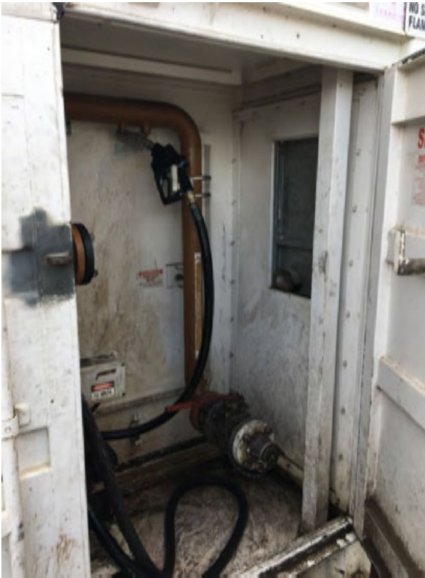
Photograph B.4 Bundled diesel above ground storage unit (June 2018)
