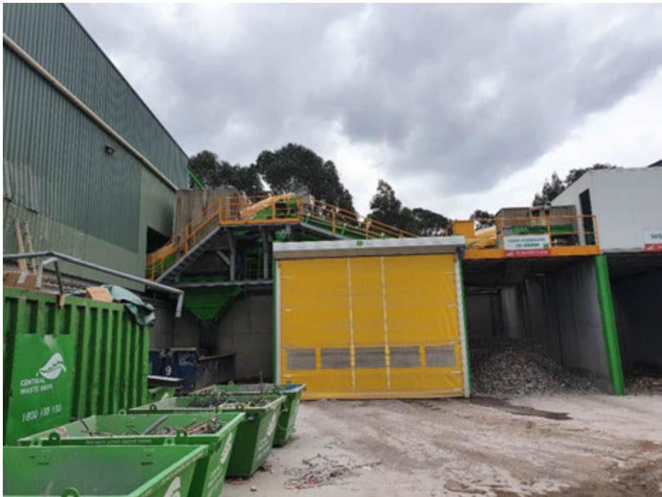
Photograph 6 – (8 Styles St) Entry point conveyor for waste processing line. Raw waste enters covered area where it is separated by mechanical processes with some hand processing. Bays are situated below where various sorted products are dropped out from the processing line.
