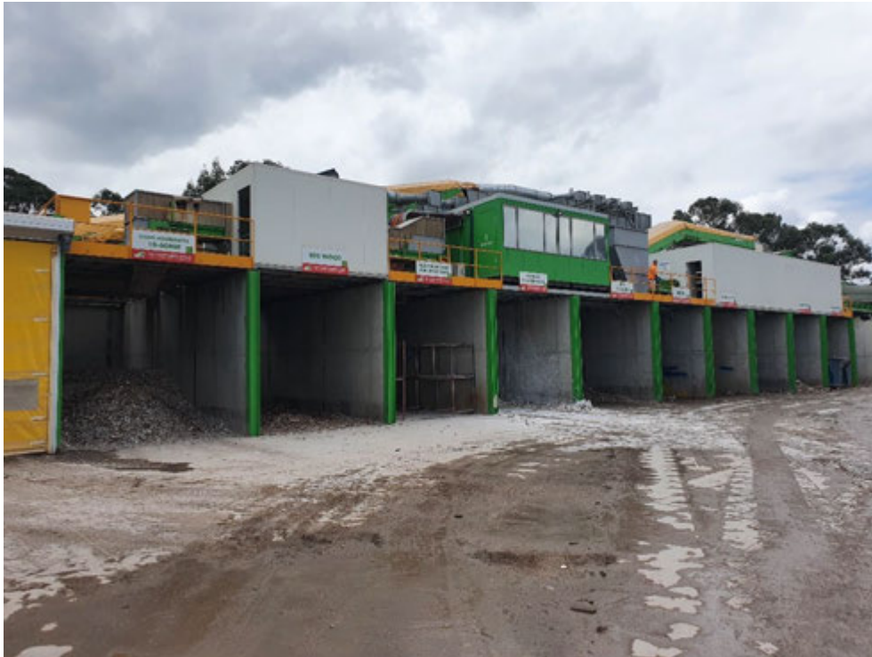
Photograph 7 – (8 Styles St) Storage bays for processed waste located under the processing conveyor.
