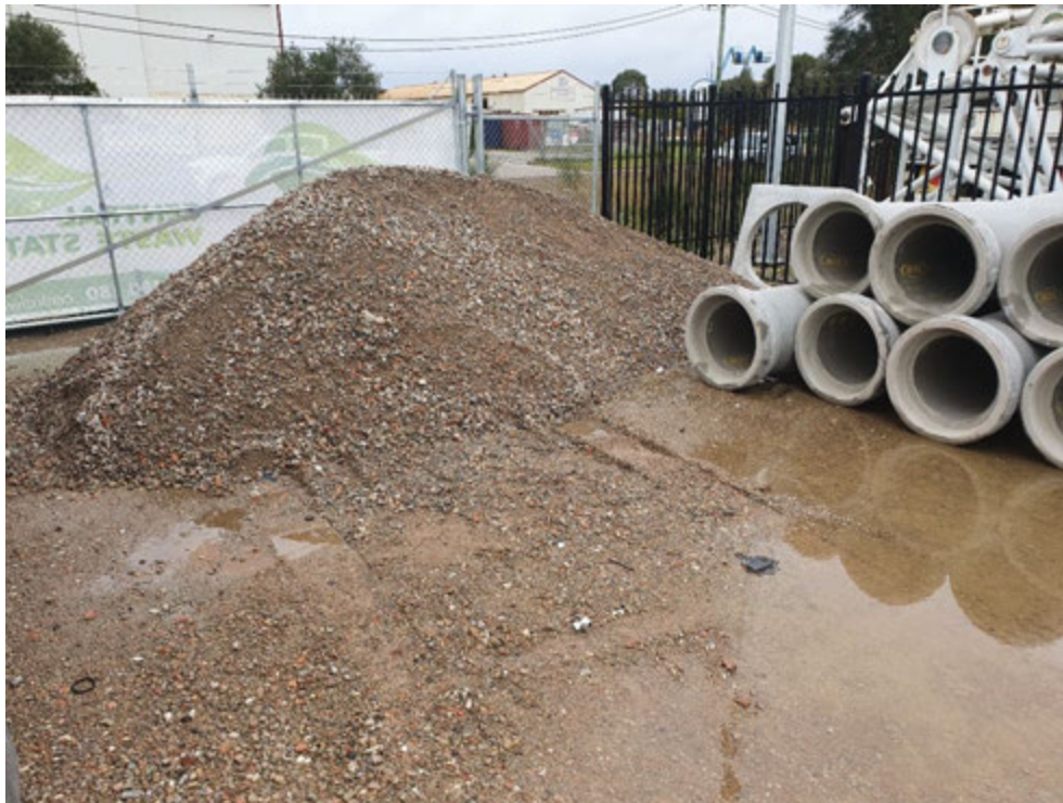
Photograph 5 – Imported recovered aggregate generated by CWS which was used as a hardstand cover for the site. Surplus material was stored in a minor quantity in 2 locations.
