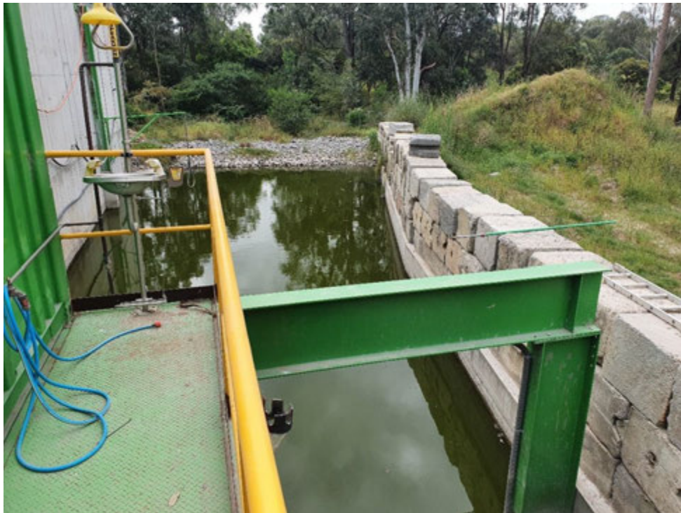
Photograph 8 – (8 Styles St) Dedicated water storage dam which collects surface flows. Picture taken from dosage and pump station located above the dam.
