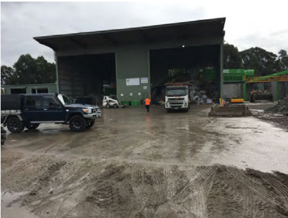
Photograph B.9 Sealed and unsealed boundary in front of sorting shed (June 2018)
