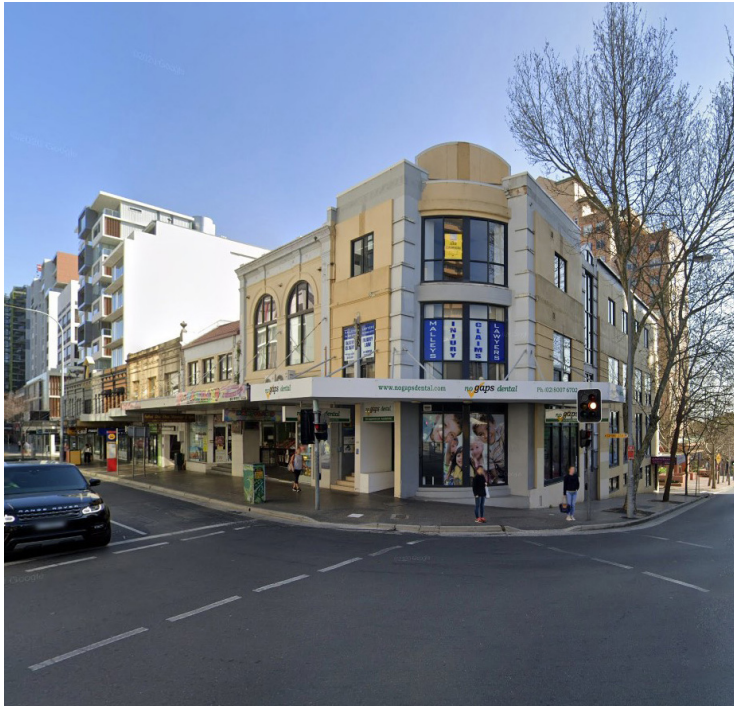
South-Eastern corner of the site from the corner of Oxford and Newland Street
