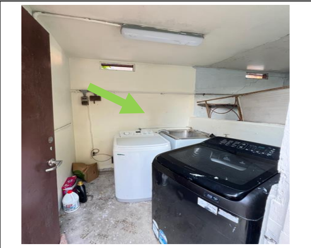
Photograph 8 (20.06.24): Representative yellow paint system, external backyard laundry shed walls, Sample ID: Same as 4-LP8 (0.03 % w/w)
