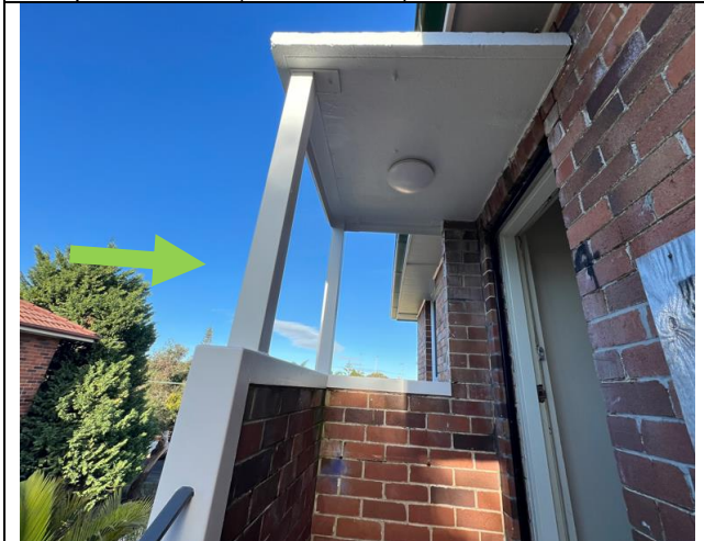
Photograph 9 (20.06.24): Representative photo of white paint system, external porch area, Sample ID: 4-LP6 (<0.01 % w/w)
