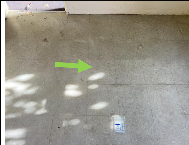
Photograph 13 (20.06.24): Representative photo of vinyl tiles on the internal kitchen floor, Sample ID: 4-A2 (NAD).
