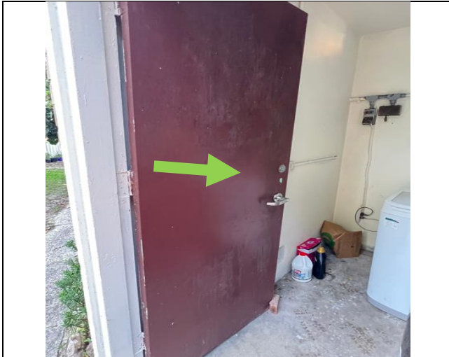
Photograph 7 (20.06.24): Representative photo of brown paint system, external backyard laundry shed door, Sample ID: 4-LP5 (< 0.01 % w/w)
