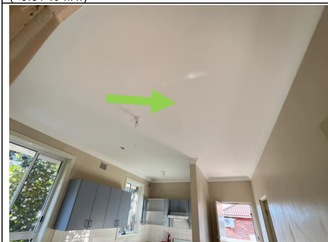
Photograph 11 (20.06.24): Representative photo of white-coloured plasterboard, internal kitchen and hallway ceiling, Sample ID: 4-A1 (NAD)
