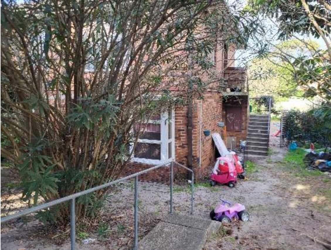
Image 2.2.11 Photograph taken facing south showing a portion of the two-storey building located at 195 Fitzgerald Avenue.
