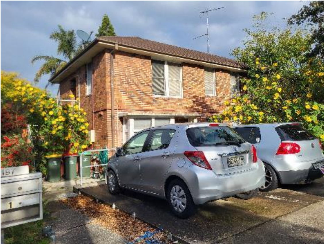
Image 2.2.10 Photograph taken facing south-west showing a portion of the two-storey building located at 197 Fitzgerald Avenue.
