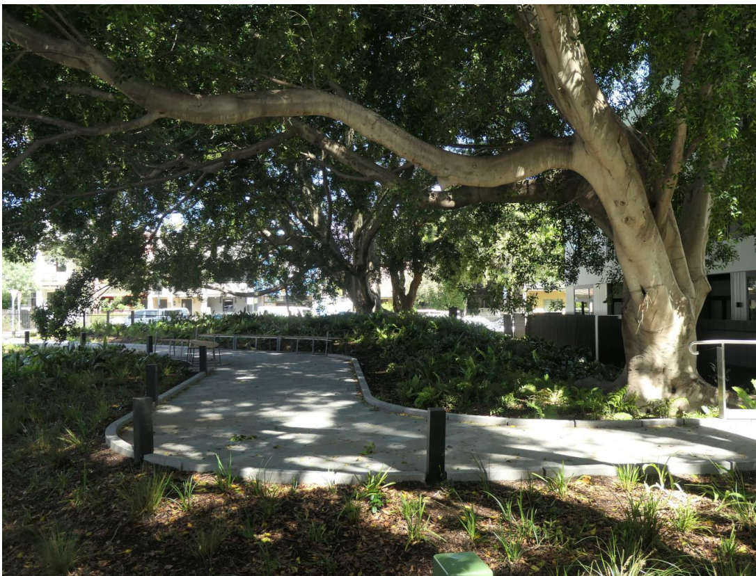
Figure 13 – Example in Ashmore of footpath proposed under Fig tree – This is the footpath installed and finished under the Fig tree. The footpath was installed above the existing surface levels and above the existing tree roots (Photo: Arterra 06/11/21).
