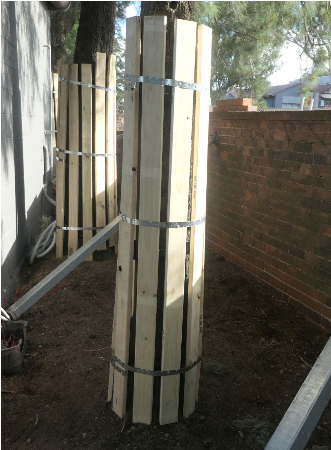
Figure 22 – Example of acceptable Trunk Protection batten installation (Photo: Arterra).
