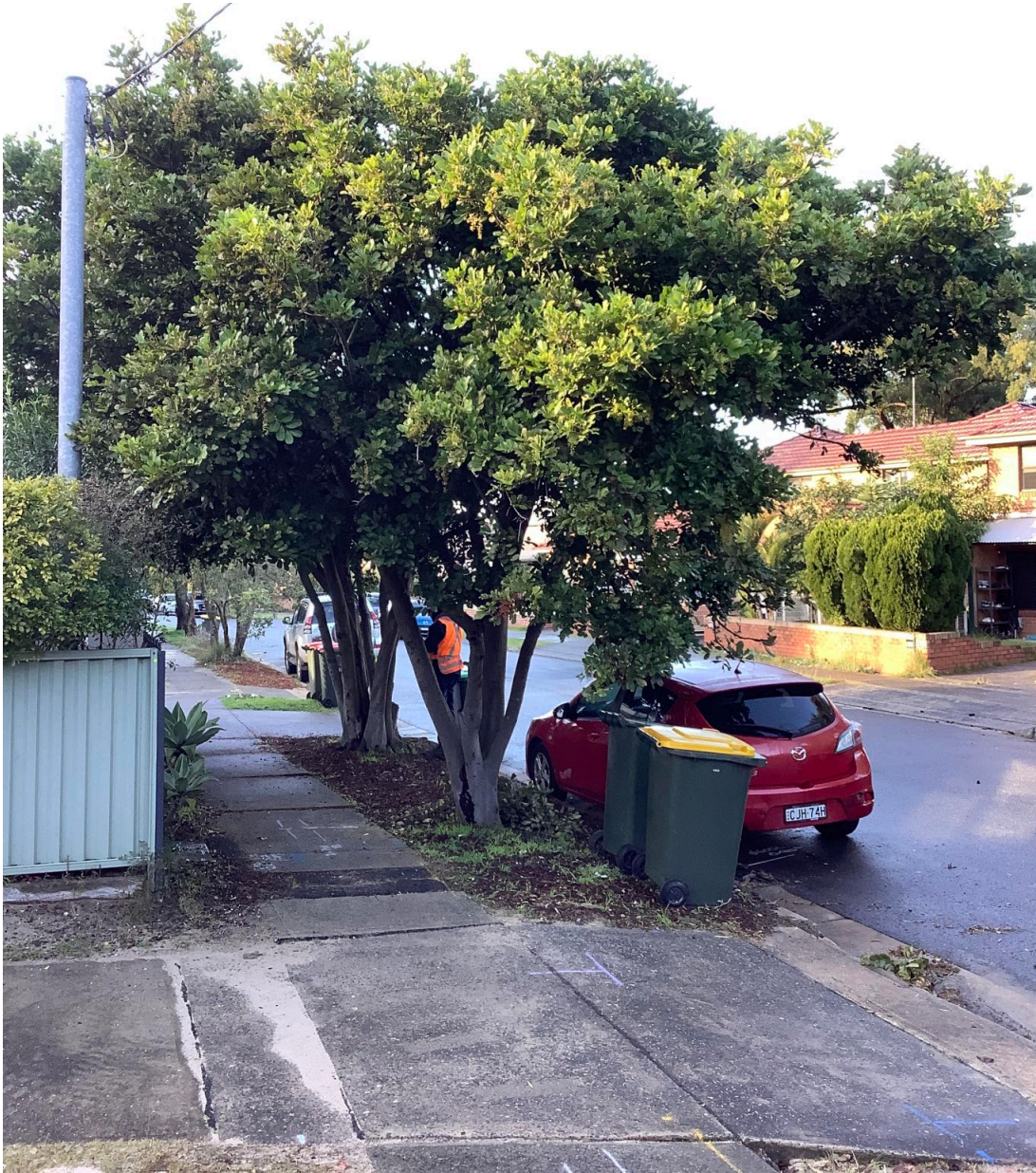
Figure 19 – Tree T02 Cupaniopsis anacardioides – Minor surface impacts expected for the construction of a new stormwater line installed non-destructively (Photo: Arterra 04/06/24).
