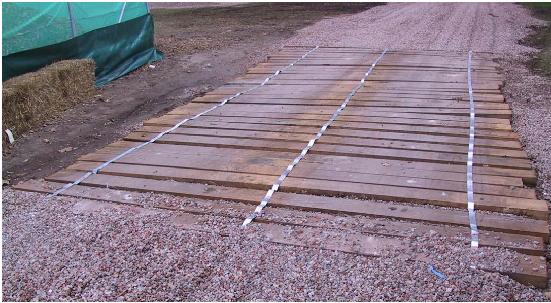
Figure 20 – Example of acceptable Tree Protection Area ground protection (Photo: Arterra).
