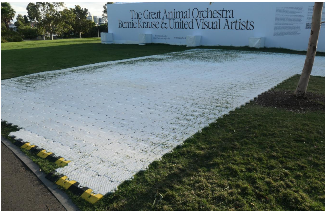
Figure 21 – Example of acceptable Tree Protection Area ground protection (Photo: Arterra).
