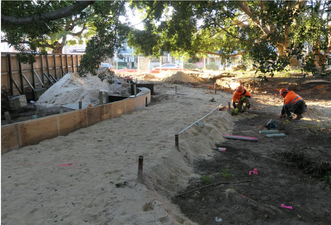
Figure 12 – Example in Ashmore of footpath proposed under Fig tree - Traditional installation of a concrete footpath on the existing ground surface was not an achievable option that protected the trees ongoing health. To protect the existing Fig tree and the above ground roots, the area under the trees was back filled with nominally 300-400mm of sandy soil. This covered over and protected the existing roots and created a level pad to install the concrete pathway without impacting on or compromising the existing roots (Photo: Arterra 20/07/20).
