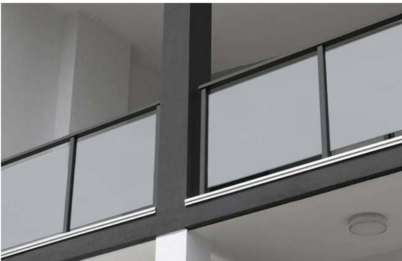
METAL FRAMED SOLID PANEL BALUSTRADE
