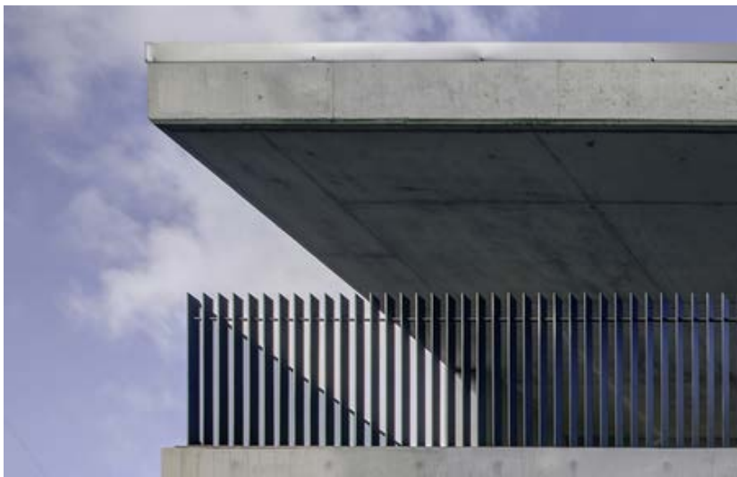
STEEL PAINT ON METAL BALUSTRADES
