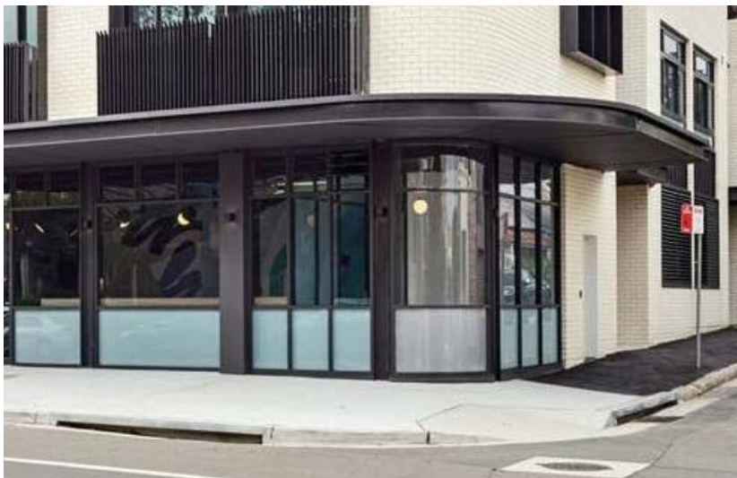
METAL CLAD STEEL FRAME AWNING
