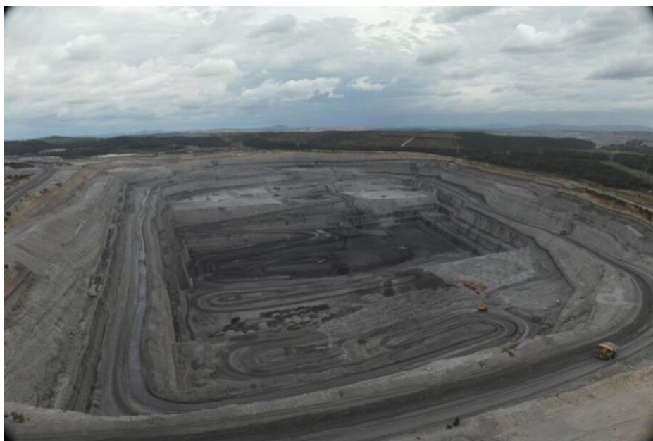
Figure 4-1 United Open Cut operations in December 2025
