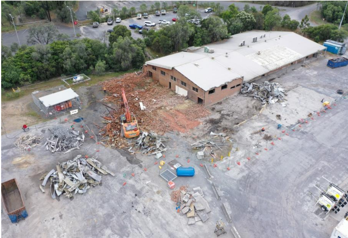
Figure 6-5 North MIA demolition in progress. Ferrous waste separated from others to be sent for offsite recycling.
