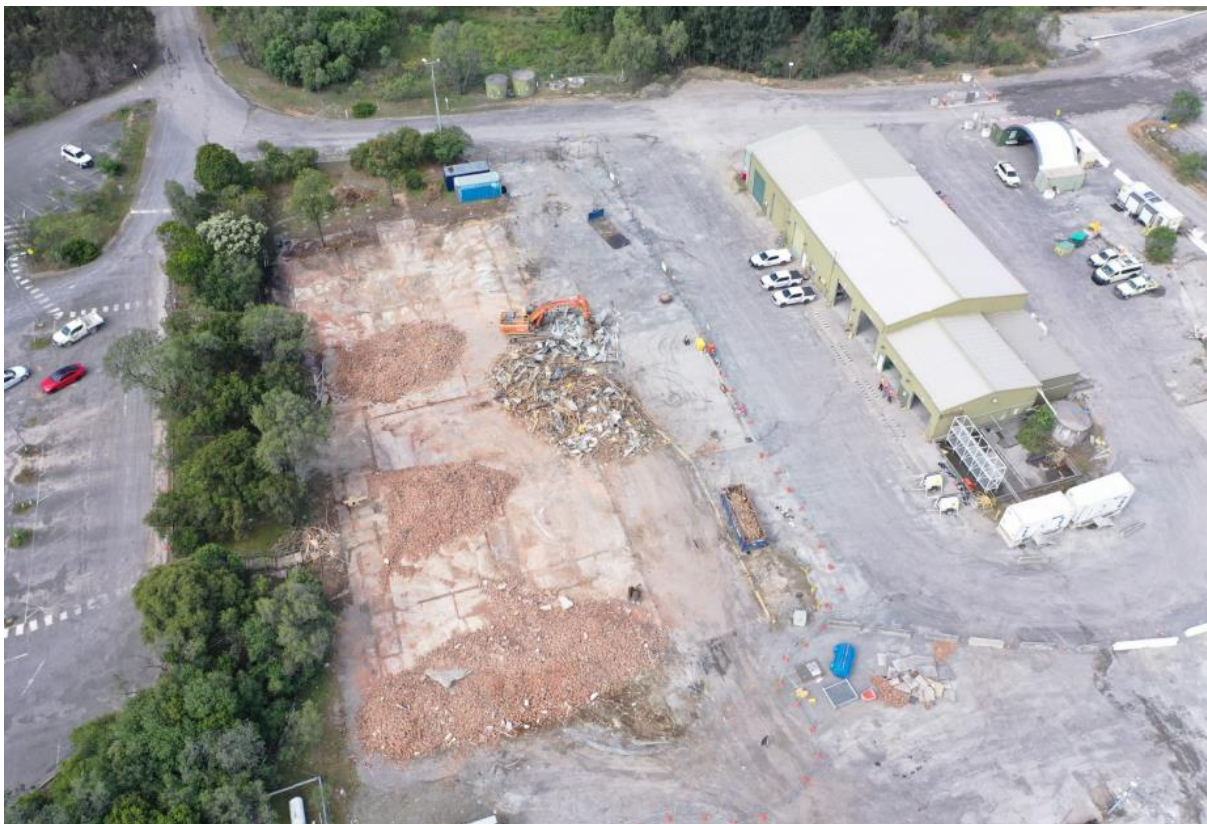
Figure 6-6 North MIA demolished and waste being prepared for disposal/recycling.
