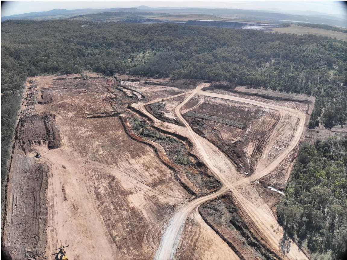
Figure 7-26 U1 Dam during construction – clearing and stripping
