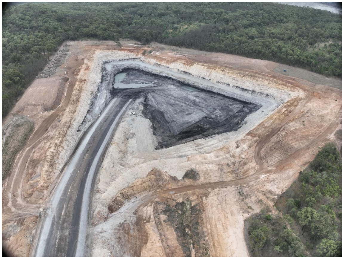
Figure 7-27 U1 Dam during construction – mining
