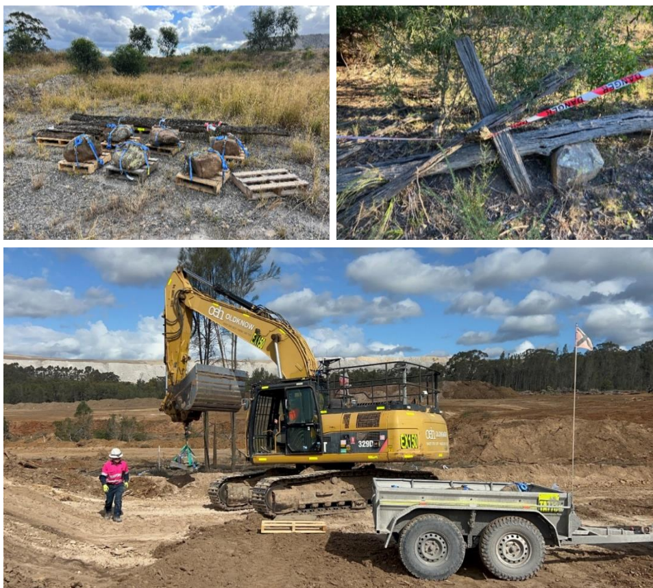
Figure 6-4 Photos taken throughout the process of the dog-leg fence salvage, including the salvaged pieces, a section of the dog leg fence in-situ marked for salvage and the process for the salvage of 6 sandstone blocks.
