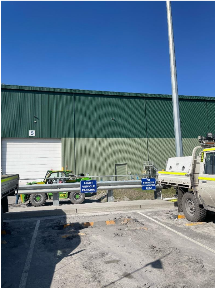
Plate 7 Cladding on UWJV workshop to reduce visual contrast from external views
