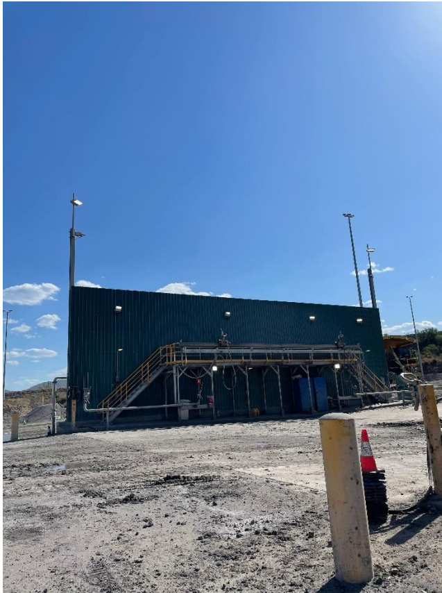
Plate 11 Fixed Lighting on Vehicle Washdown Bay
