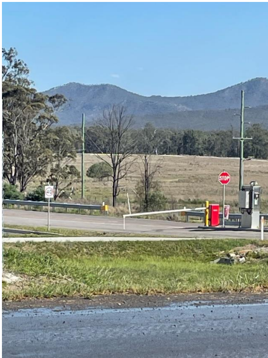
Plate 17 Security boom gate on site access
