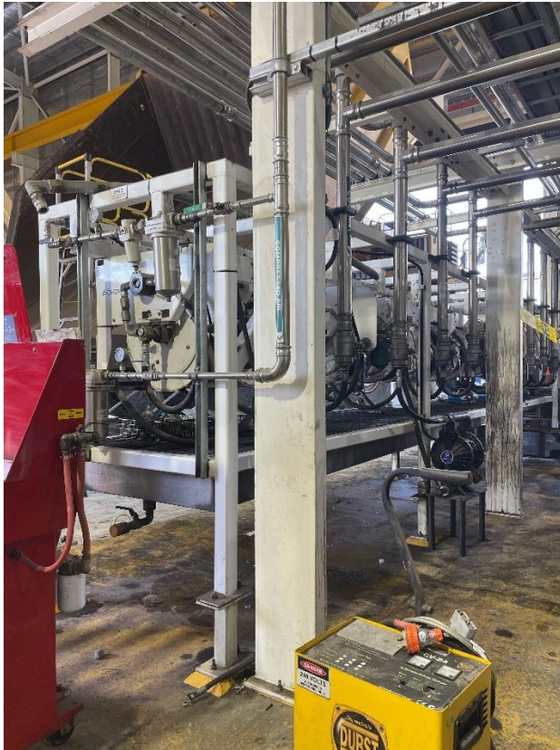
Plate 3 Chemical bunding inside workshop
