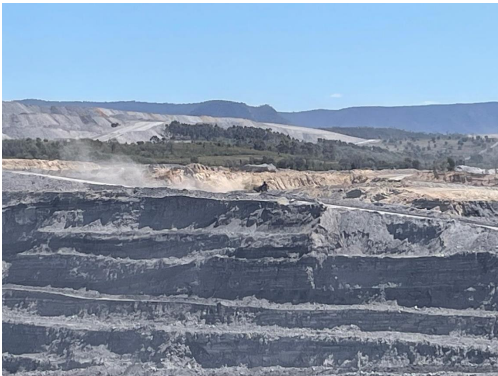
Plate 8 Localised dust emissions from excavator operations sighted during site inspection
