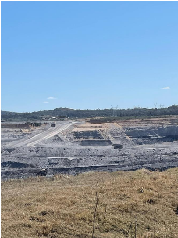
Plate 9 Haul road dust emissions management observed during site inspection
