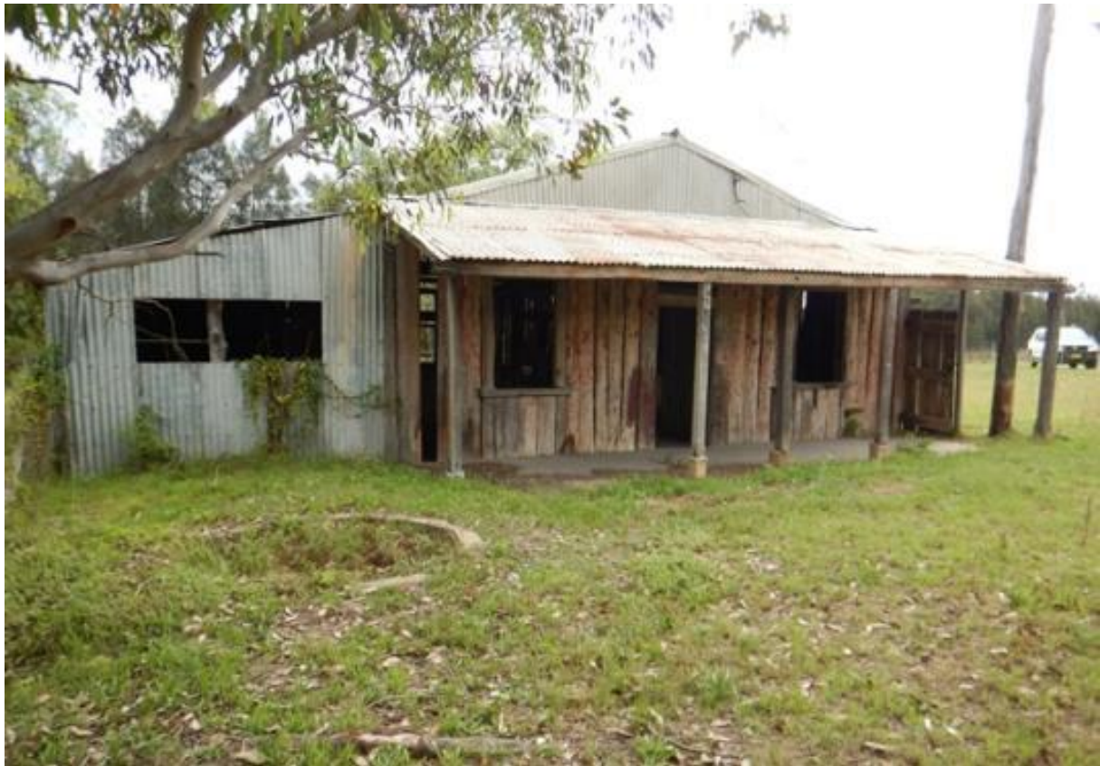
Plate 7-6: View to West of Shearing Shed Note, in-ground cistern in front of shed © Umwelt, 2015
