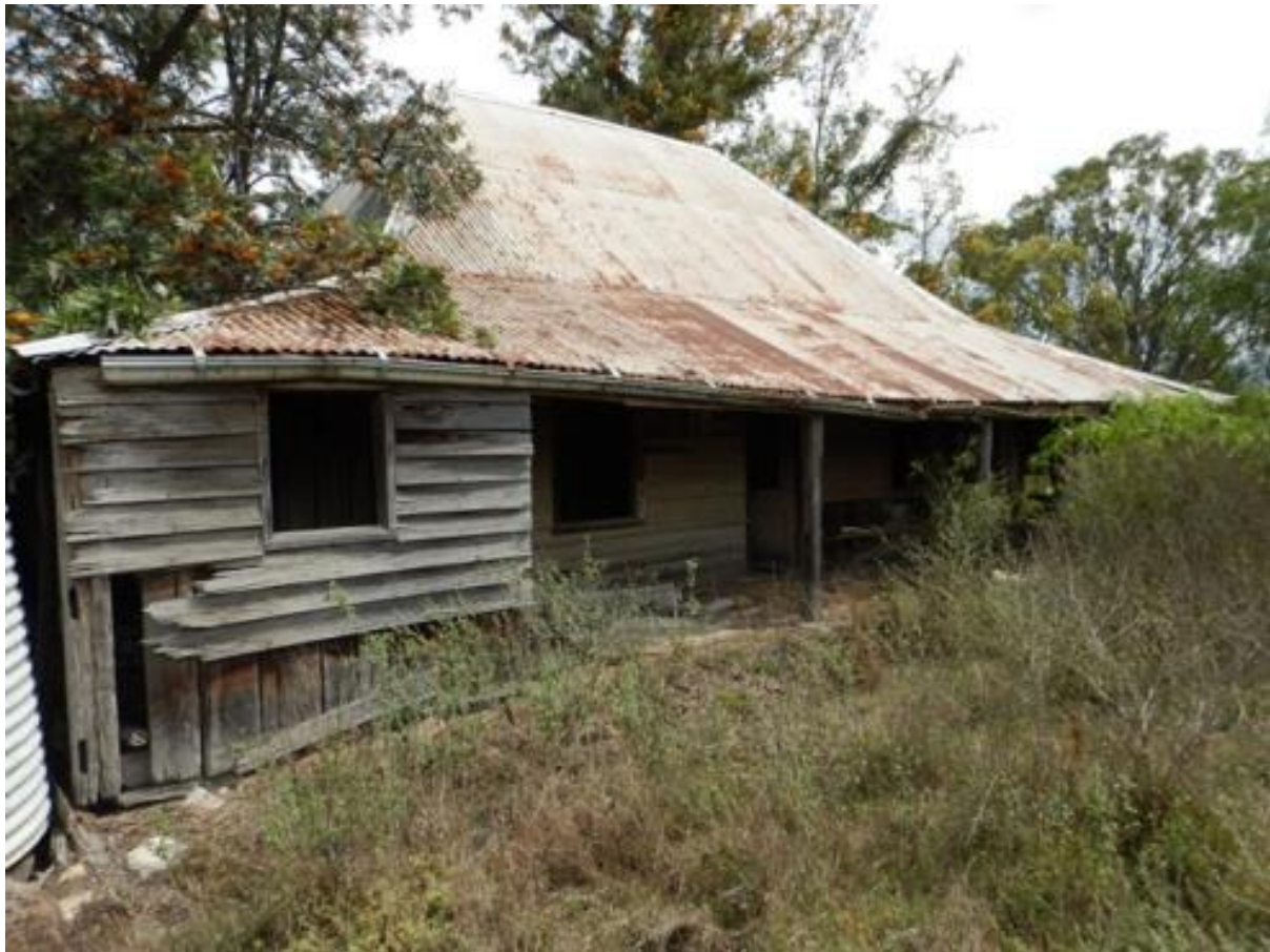
Figure 3-11 View to South-West Showing Front Elevation of Cottage
