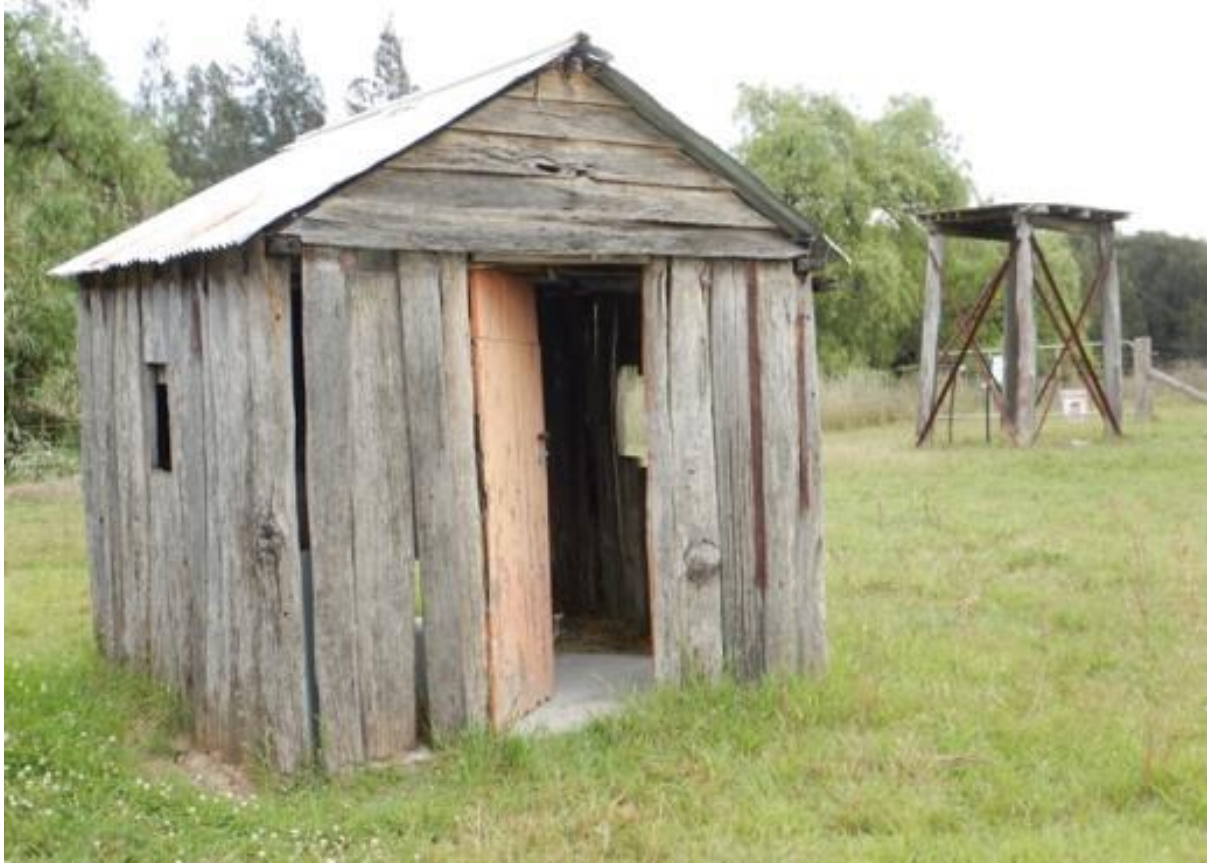
Figure 3-6 View to West of Creamery and Timber Tank Stand Note, new concrete slab of creamery
