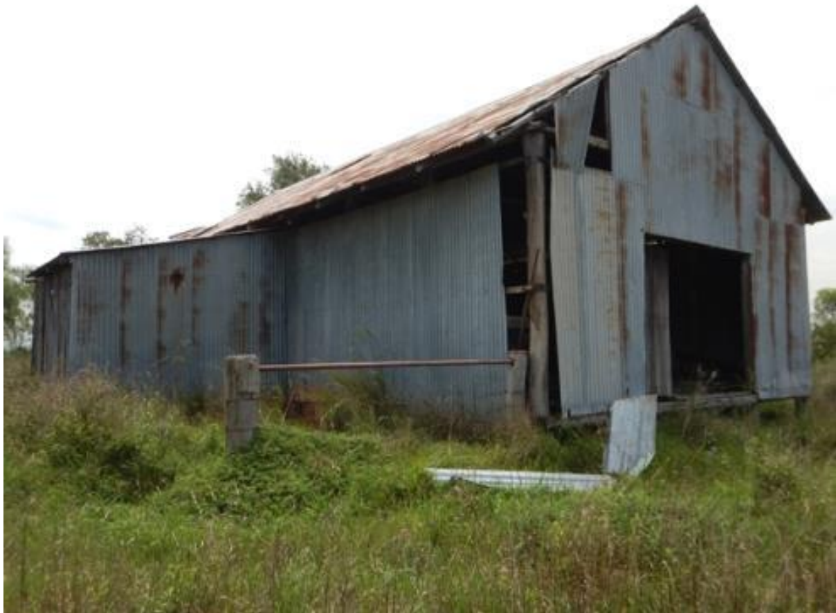
Figure 3-9 View to North of Montrose Property Shearing Shed
