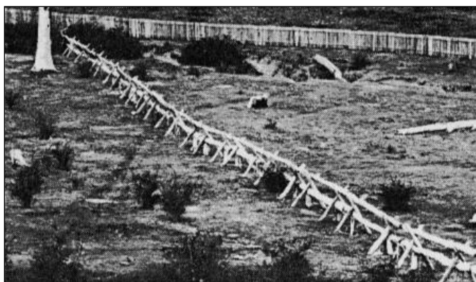
Dog-leg fence on 'A cleared property in Southern New South Wales, c. 1880'. (Detail from Merritt & O'Brien 1985, p. 5)
