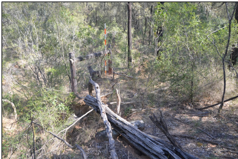
[Image 12] DSC_1046 Pic 78. Junction of fences in the southern end of the boundary between Portion 107 and 128. The end assembly at the ranging pole is on the lip of the step creek bank ~ 6 high. Wire was used across the creek. A stone block and bottom log in the foreground are part of the north-south fence, but the dog-leg fence running east is out of the image.
