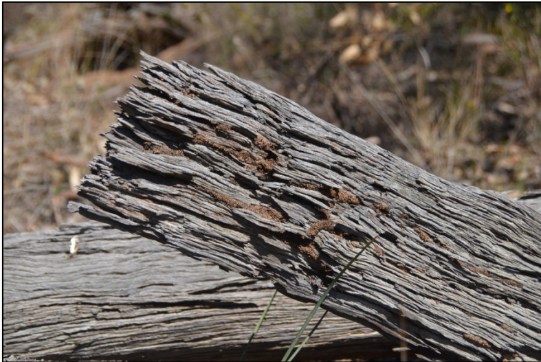
[Image 18] DSC_1011 Pic 42. Termite tracks on split dog-leg.
