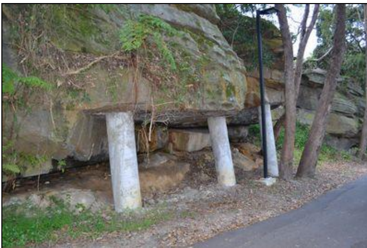
Photograph 3: Facing east and looking at AHIMS 45-6-1974 and AHIMS 45-6-1975 which are now supported by concrete pylons.
