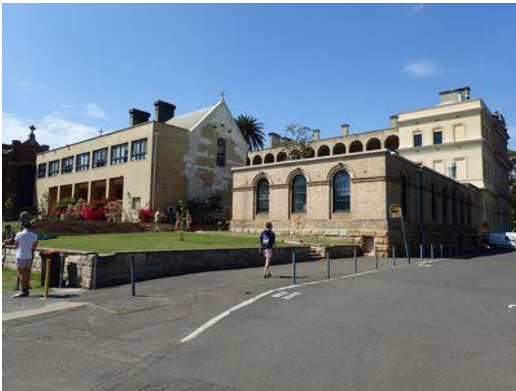
Photograph 11: Facing east and looking at the rear of the Main Building (in the background), Licona (on the right of the photo) and St Michael's House on the left of the picture.
