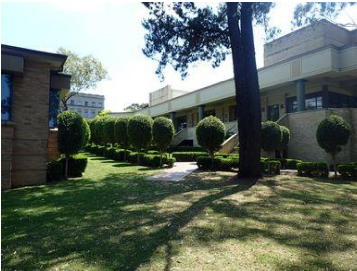
Photograph 10: Facing north west and looking toward the Wallace Building.
