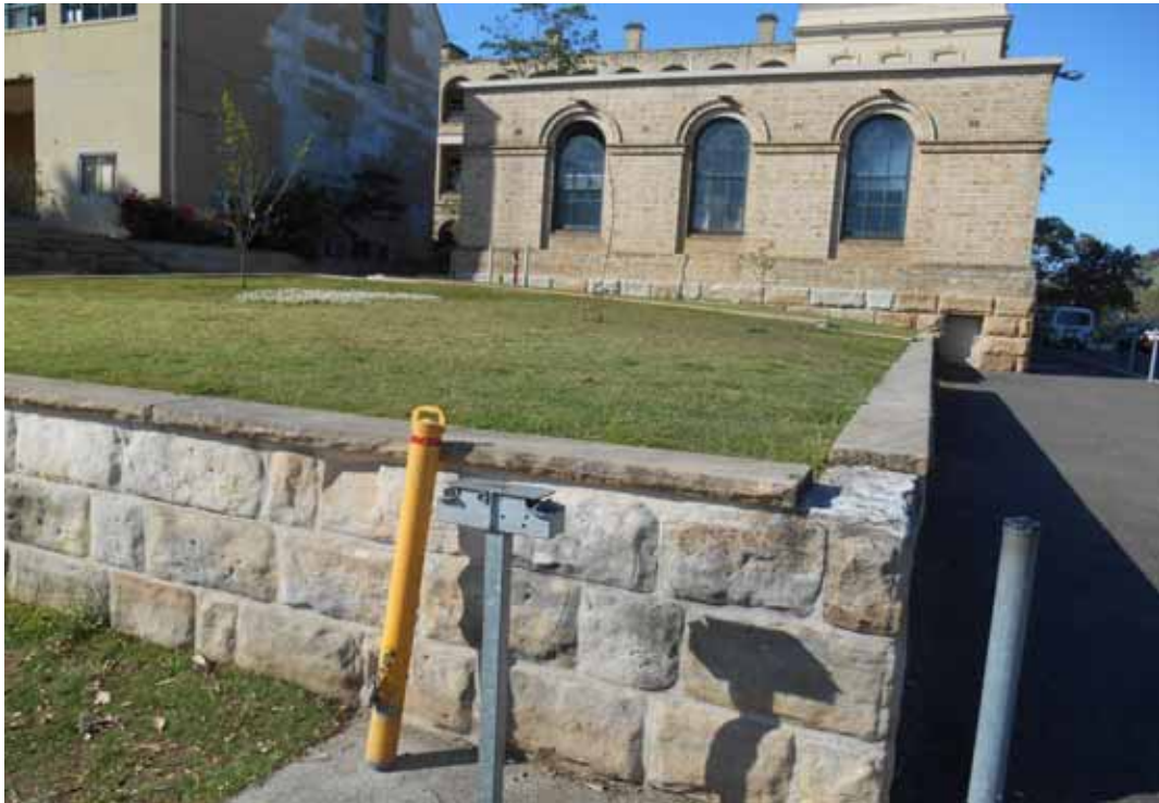
Photograph 1 - Retaining wall near Saint John's House
