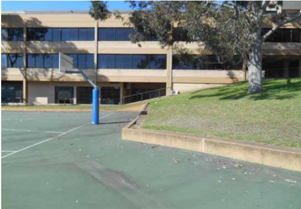
Photograph 3 - Slope and small retaining wall next to basketball courts
