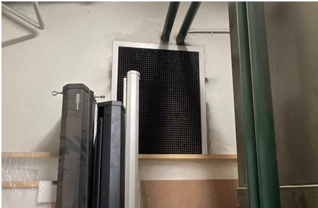
Photo F8: View Inside One of the Buildings Showing a Mesh Screen which would be Preventing Bats from entering the Building
