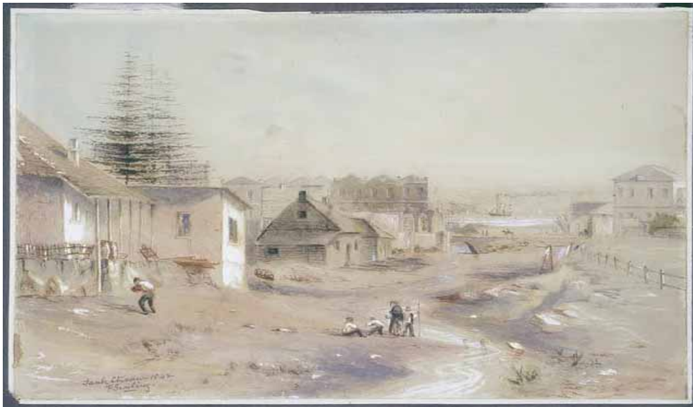
FIGURE 2-4 Garling, F. Tank Stream 1842, Mitchell Library 420.
