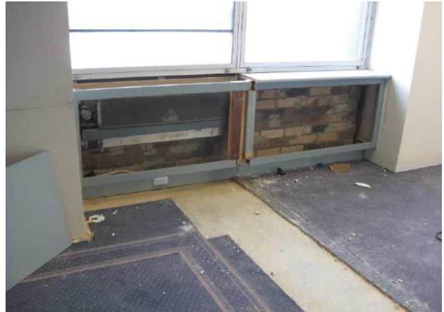
Photograph 4: Fairfax House, Level 15 plant room, metal sheeting affixed to walls and columns protecting suspected underlying friable asbestos.
