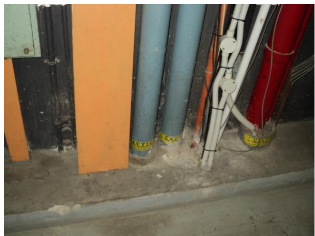
Photograph 6: Fairfax House, Level 15 plant room, suspected ACM cable and pipe penetration packing.
