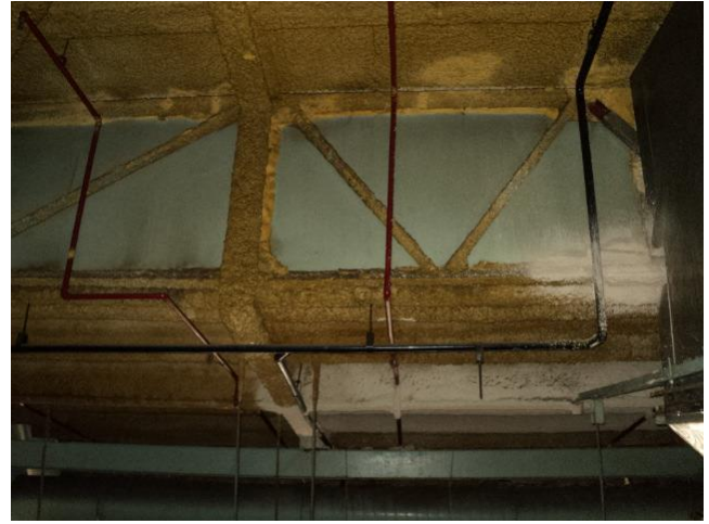
Photograph 8: Fairfax House, Level 15 plant room, exposed (sealed) friable asbestos to underside of the roof and on structural steel.
