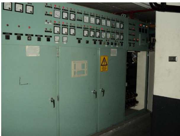
Photograph 5: Fairfax House, Level 15 plant room, suspected ACM electrical backing boards.
