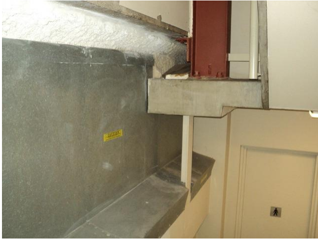
Photograph 7: Fairfax House, Level 14-15 south west fire stairs, exposed (sealed) friable ACM to the ceiling and partially covered friable ACM with sheet metal.
