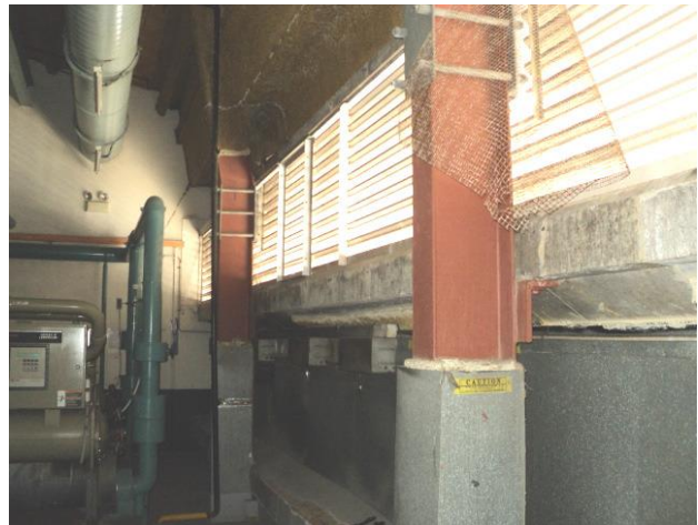
Photograph 6: Fairfax House, Level 15 plant room, suspected ACM cable and pipe penetration packing.
