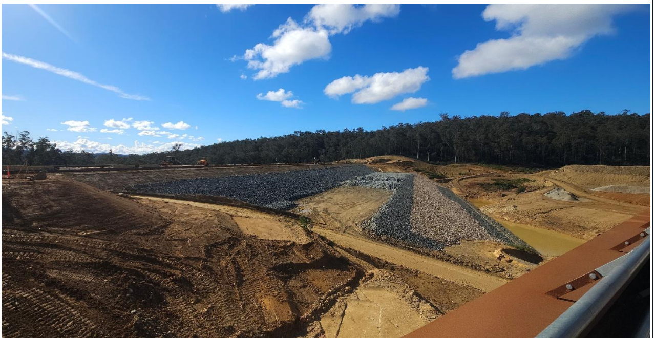
Plate 6 Construction footprint facing north from Tower Access Bridge: Water storage embankment, and sediment basin
