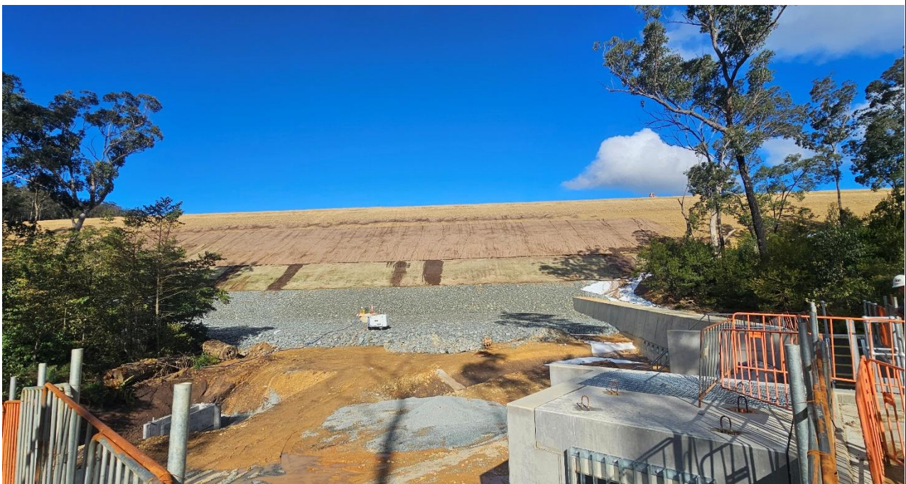
Plate 10 Construction footprint facing south-west downstream of water storage embankment, including outlet valve pit
