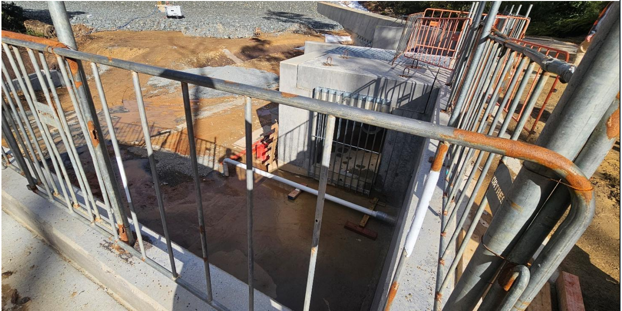
Plate 11 Outlet valve pit downstream of water storage embankment
