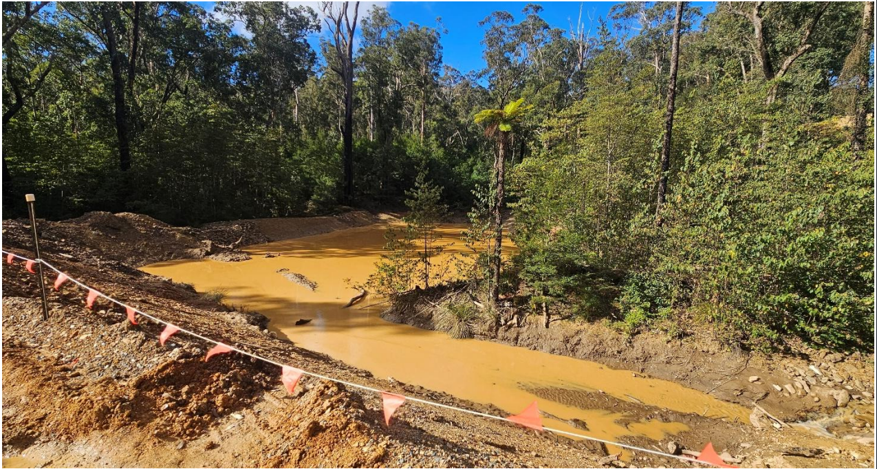
Plate 9 Construction footprint facing north-east downstream of water storage embankment
