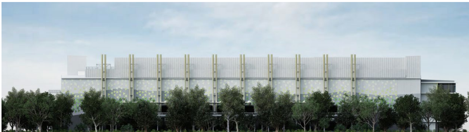
Figure 9 | Southern and Eastern façades
