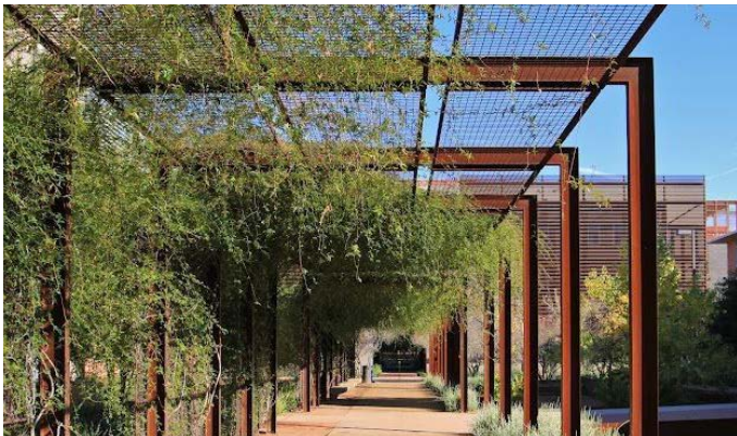
Shade structures incorporating trailing plants
