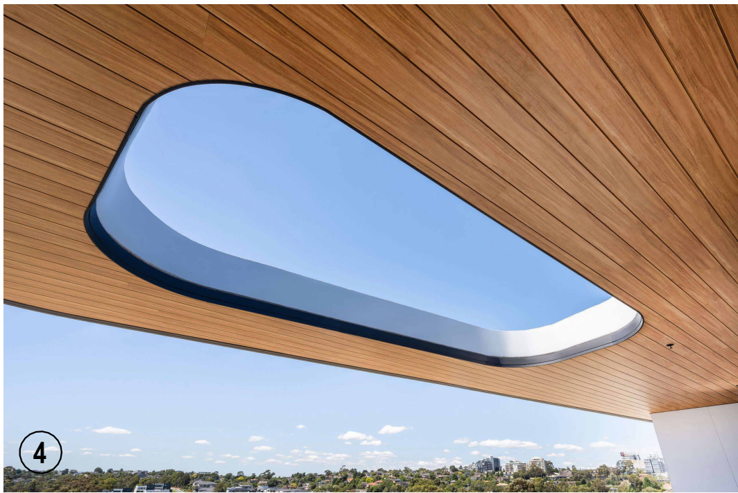
TIMBER PANEL SOFFIT
