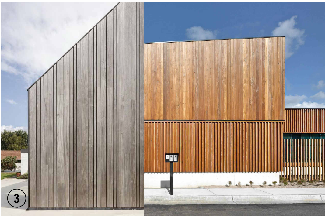
WEATHER TIMBER BOARD CLADDING
