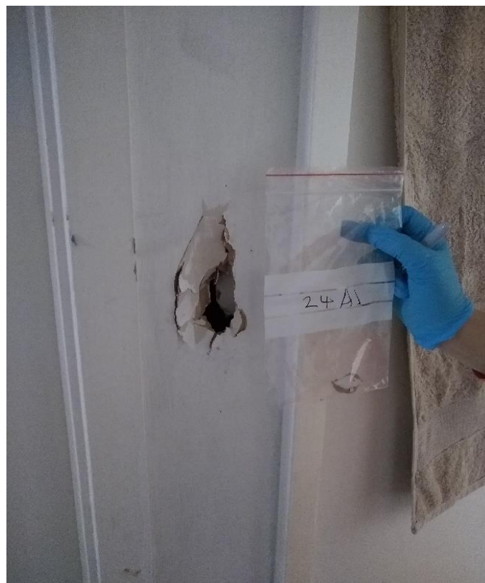
Photo 12: Building 24, interior, wall sheeting in corridor of house, plaster sheeting, sample 24A2, no asbestos detected by analysis.
