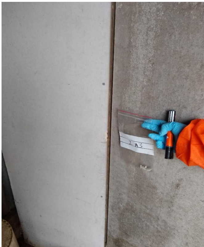
Photo 3: Building 2, interior, wall sheeting, fibre cement sheeting, sample 2A3, no asbestos detected by analysis.
