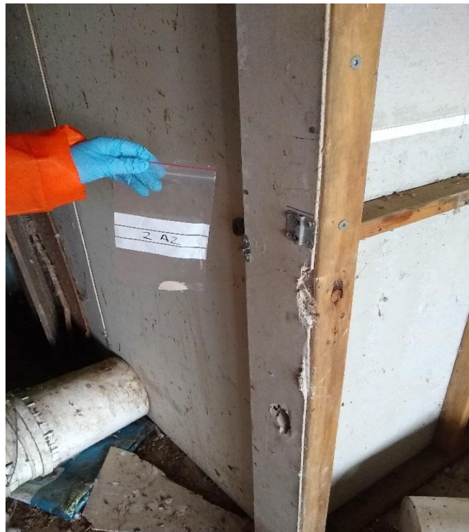
Photo 2: Building 2, interior, wall sheeting, fibre cement sheeting, sample 2A2, no asbestos detected by analysis.
