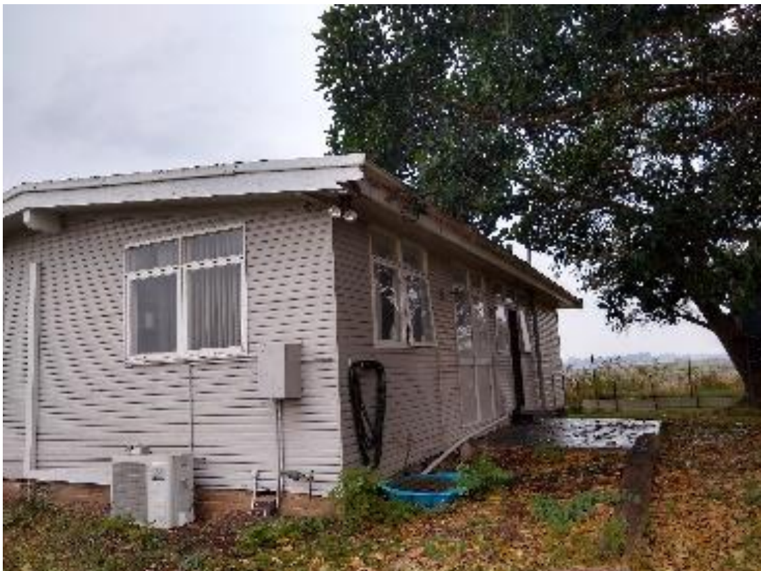
Photo 64: Building 24, ceiling cavity, throughout ceiling cavity, insulation generally, SMF (suspected)
