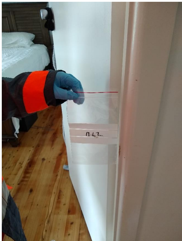
Photo 30: Building 11, interior, paint off timber door frame to bedroom in north eastern portion of house, white paint, sample 11L2, no lead paint(s) identified
