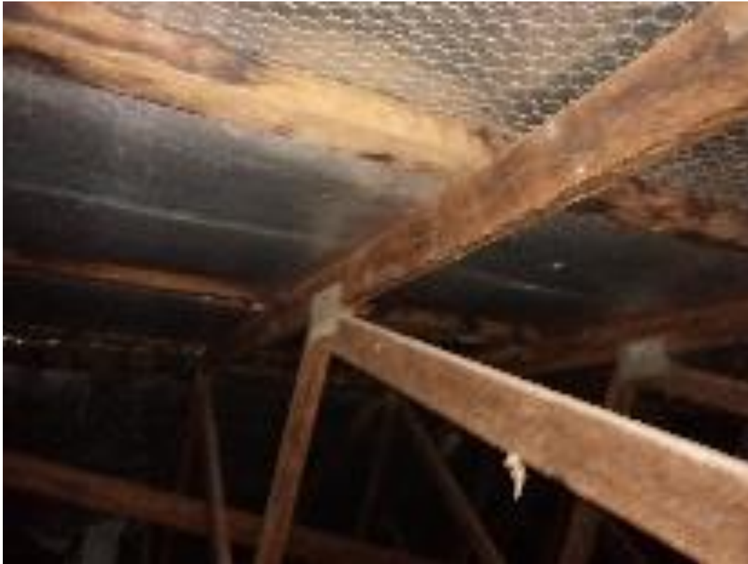
Photo 53: Building 25, manhole in central western portion of house, throughout, settled dust, sample 25D2, lead concentration <0.5 mg/m2
