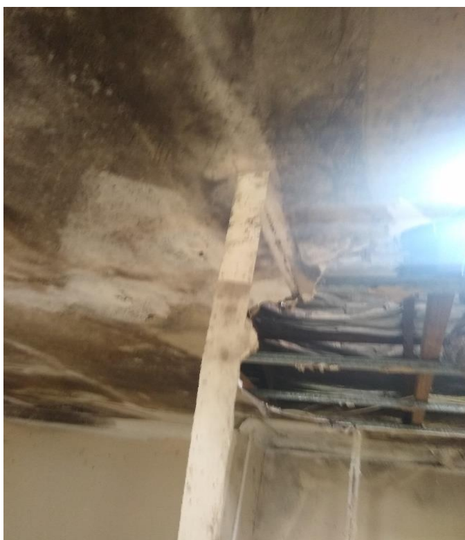
Photo 4: Building 4, interior, ceiling sheeting, plaster sheeting, sample 4A1, no asbestos detected by analysis (SMF detected).
