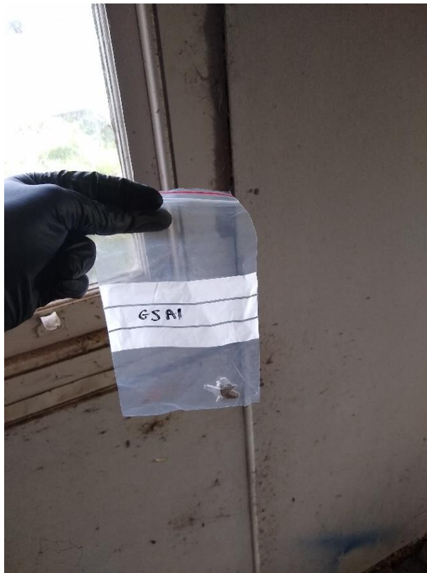
Photo 26: Building GS, interior, sheeting from walls in south western portion of garage structure, fibre cement sheeting, sample GSA1, no asbestos detected by analysis.
