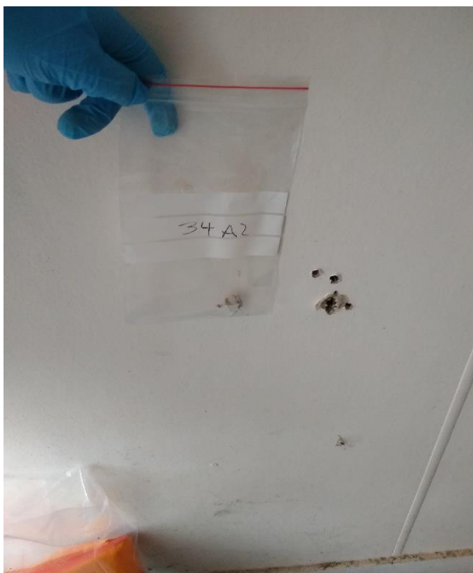
Photo 18: Building 34, interior, sheeting from wall, fibre cement sheeting, sample 34A2, no asbestos detected by analysis.
