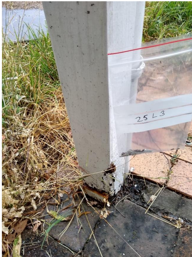
Photo 38: Building 25, exterior, paint off timber post on eastern side of house, white paint, sample 25L3, no lead paint(s) identified
