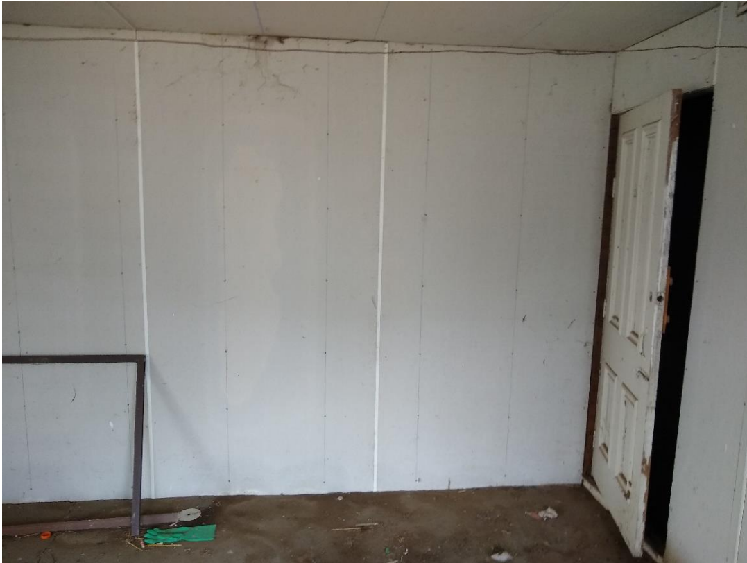
Photo 27: Building GS, interior, sheeting from walls in north eastern portion of garage structure, fibre cement sheeting, sample GSA2, no asbestos detected by analysis.
