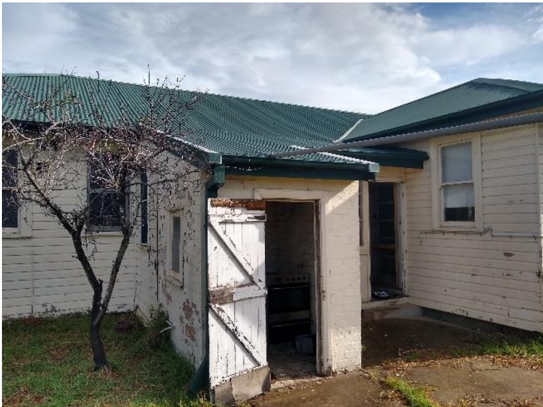
Photo 22: Building HS, exterior, sheeting from eaves, fibre cement sheeting, sample HSA1, no asbestos detected by analysis.
