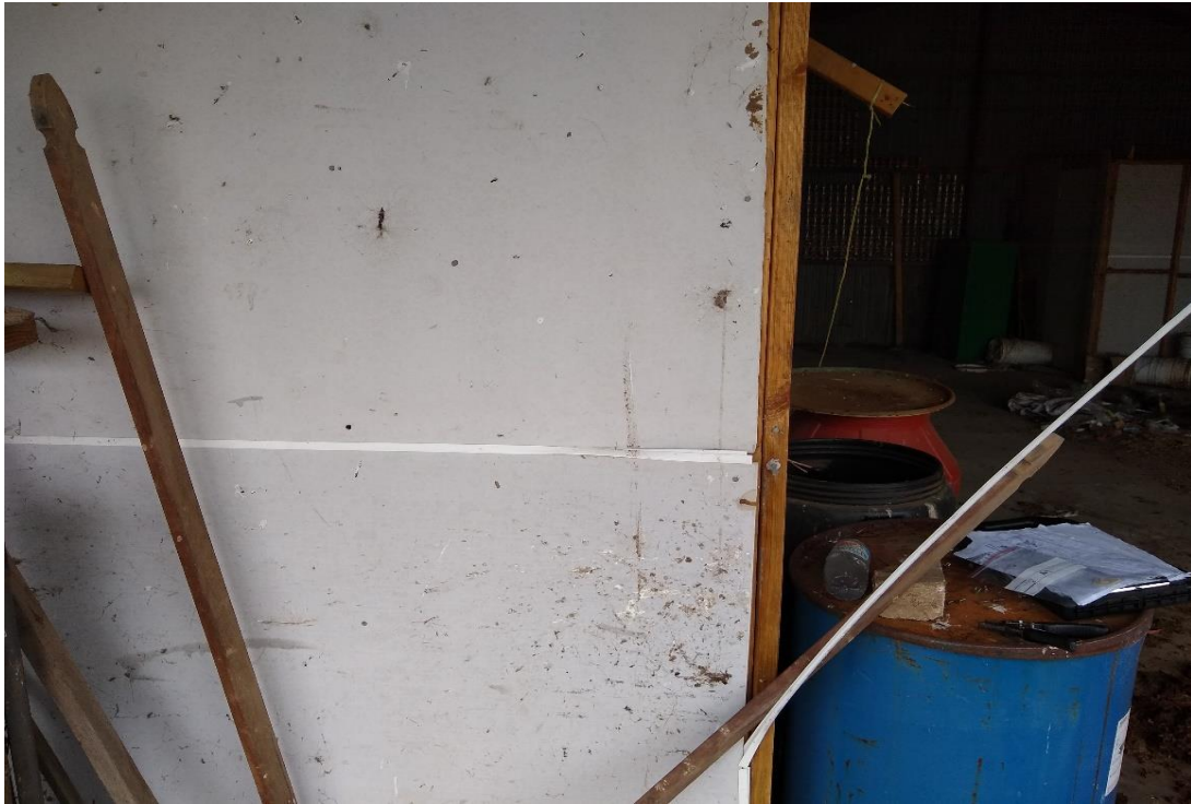
Photo 1: Building 2, interior, wall sheeting, fibre cement sheeting, sample 2A1, no asbestos detected by analysis.
