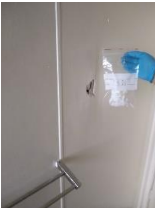
Photo 51: Building 24, wall cavity in central portion of house, throughout, settled dust, sample A4D1, lead concentration <0.5 mg/m2
