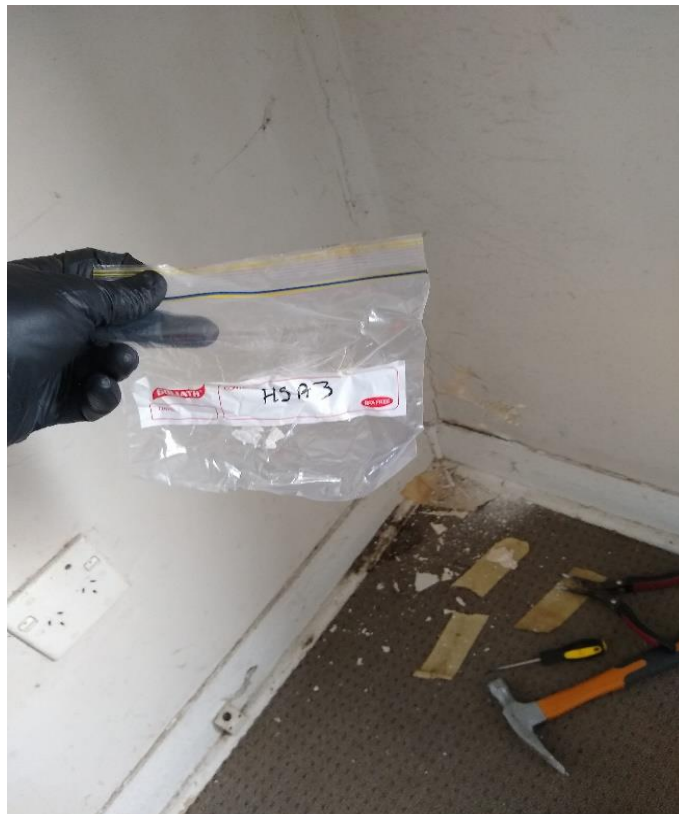
Photo 24: Building HS, interior, sheeting from walls in south western portion of house, plaster sheeting, sample HSA3, no asbestos detected by analysis.
