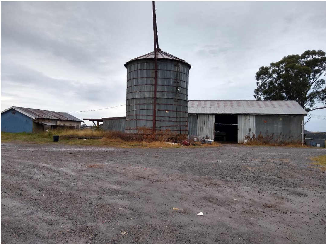
Photo 70: Structure 16 (Silo), no hazardous building materials identified
