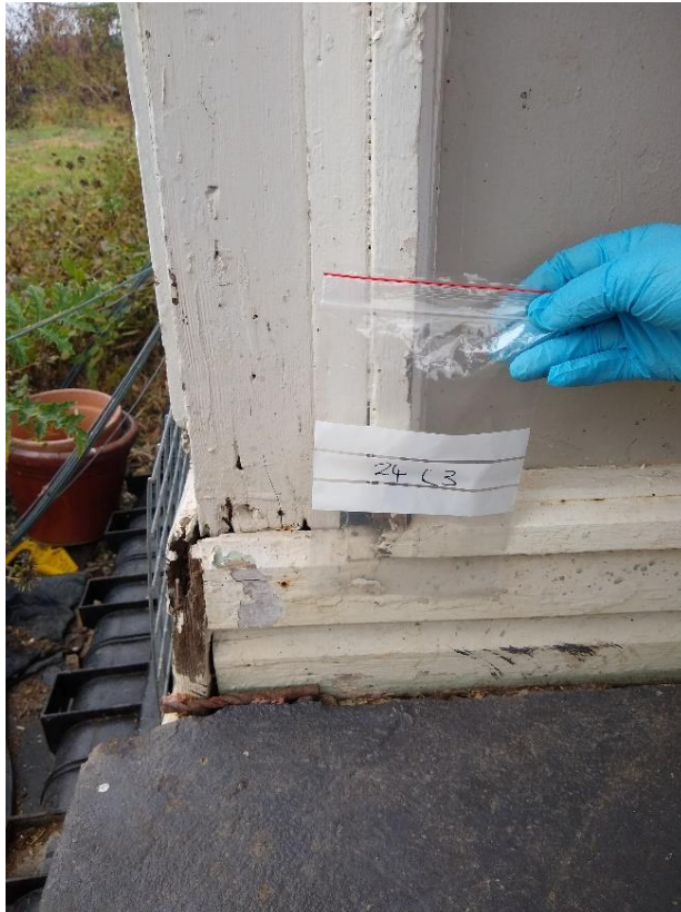
Photo 35: Building 24, exterior, paint off timber frame of north eastern portion of house, white paint, sample 24L3, no lead paint(s) identified
