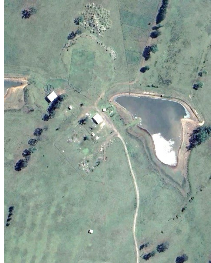
Figure 15. 2024 aerial DAH building complex dilapidation
