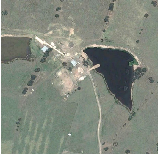
Figure 14. 2013 aerial DAH building complex dilapidation
