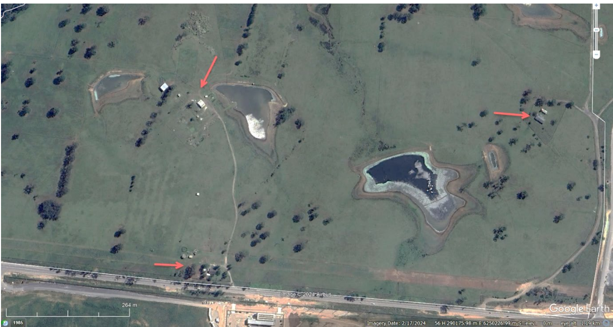
Figure 23. 2024 Air photo showing DAH buildings mostly demolished
