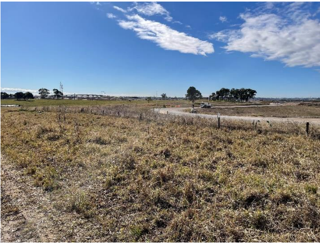
Picture 3 M12 motorway construction
