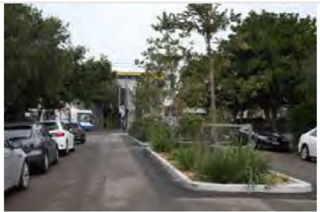
Retrofitting median street trees in Primrose Avenue, Rosebery. credit: ASPECT Studios
