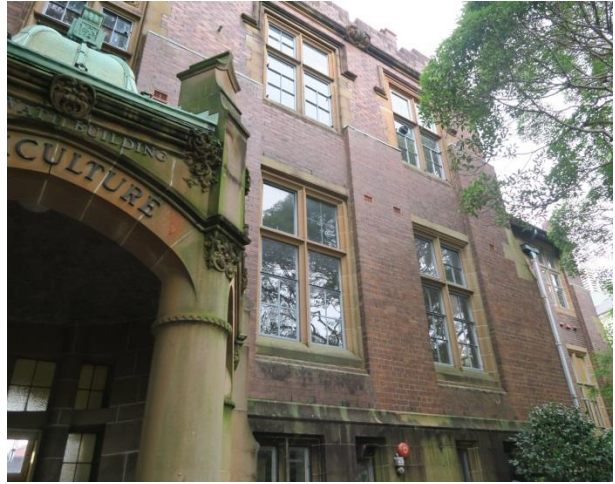
PICTURE 16 – DETAIL OF THE SOUTHERN FAÇADE SHOWING SOME OF THE MODIFIED WINDOWS
