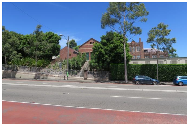
PICTURE 5 – VIEW OF THE SUBSTATION AND SIGNIFICANT PARRAMATTA ROAD FENCING
