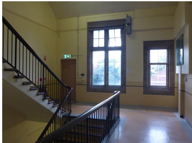
PICTURE 28 – THE STAIR HALL (VIEW NORTH) ON LEVEL 4
