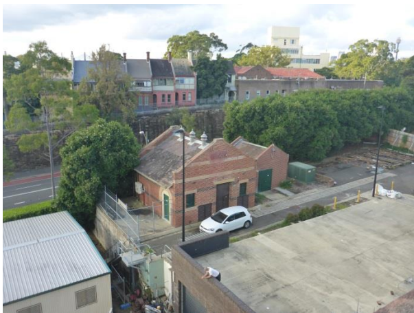
PICTURE 2 – VIEW OF SUBSTATION 54 AND SWITCH ROOM (FROM THE ROOF OF THE RD WATT). NOTE THAT THE DEMOLITION OF THE SUBSTATION IS SUBJECT TO A PREVIOUS ASSESSMENT
