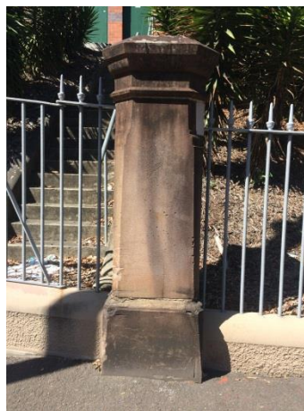
PICTURE 13 – DETAIL OF THE PARRAMATTA ROAD FENCING
