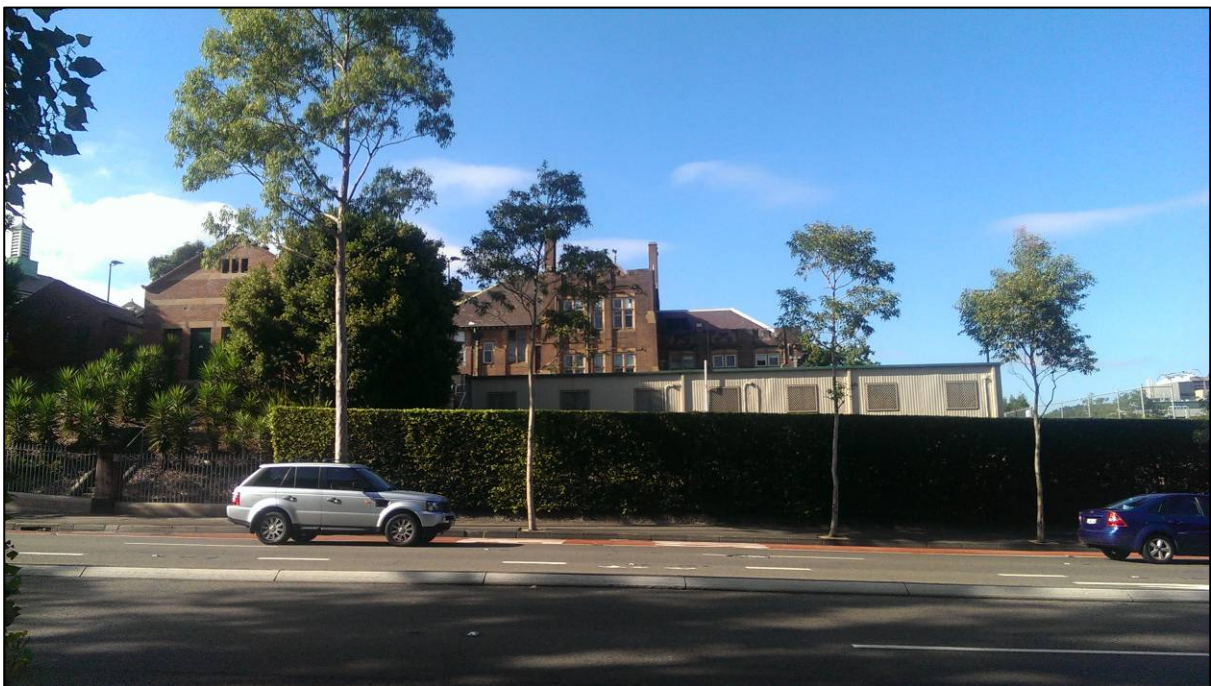
Image 8: RD Watt elevation from Parramatta Road
