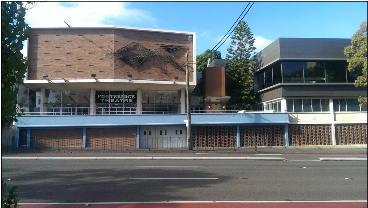
Image 7: Footbridge theatre elevation from Parramatta Road
