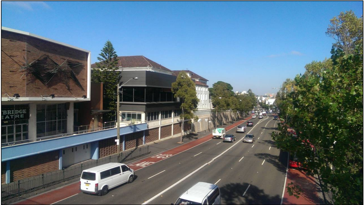
Image 5: Site view from the footbridge Parramatta Road
