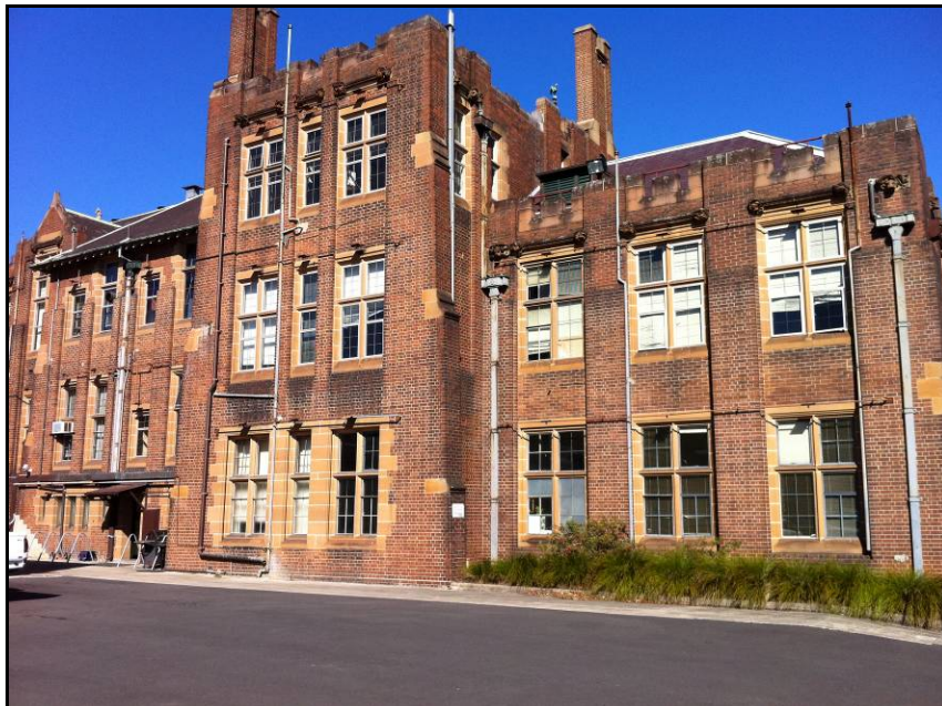
Image 2: RD Watt North elevation
