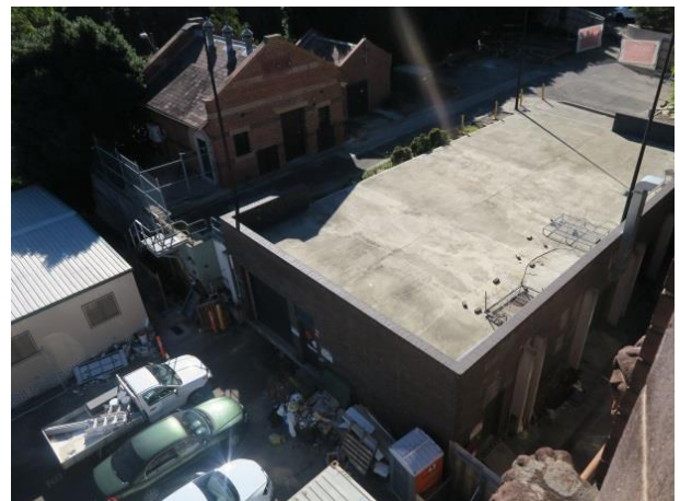
PICTURE 6 – VIEW FROM ROOFTOP TO REAR OF BUILDING.
