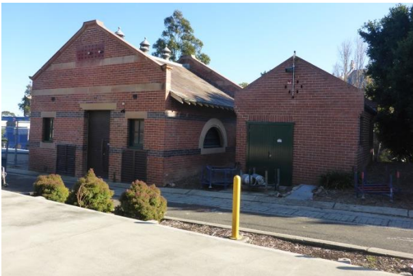
PICTURE 7 – THE SOUTHERN FAÇADE OF THE SUBSTATION, WITH THE LATER SWITCH ROOM ON THE RIGHT OF THE IMAGE.
