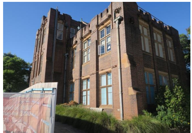
PICTURE 4 – VIEW OF THE REAR FACADE
