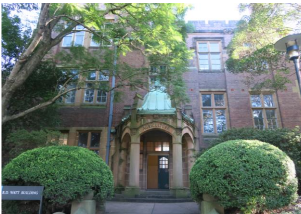
PICTURE 3 – VIEW OF THE PRINCIPAL FACADE
