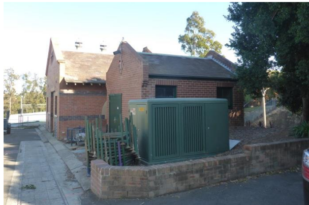
PICTURE 8 – VIEW WEST TOWARDS THE SUBSTATION AND SWITCH ROOM.
