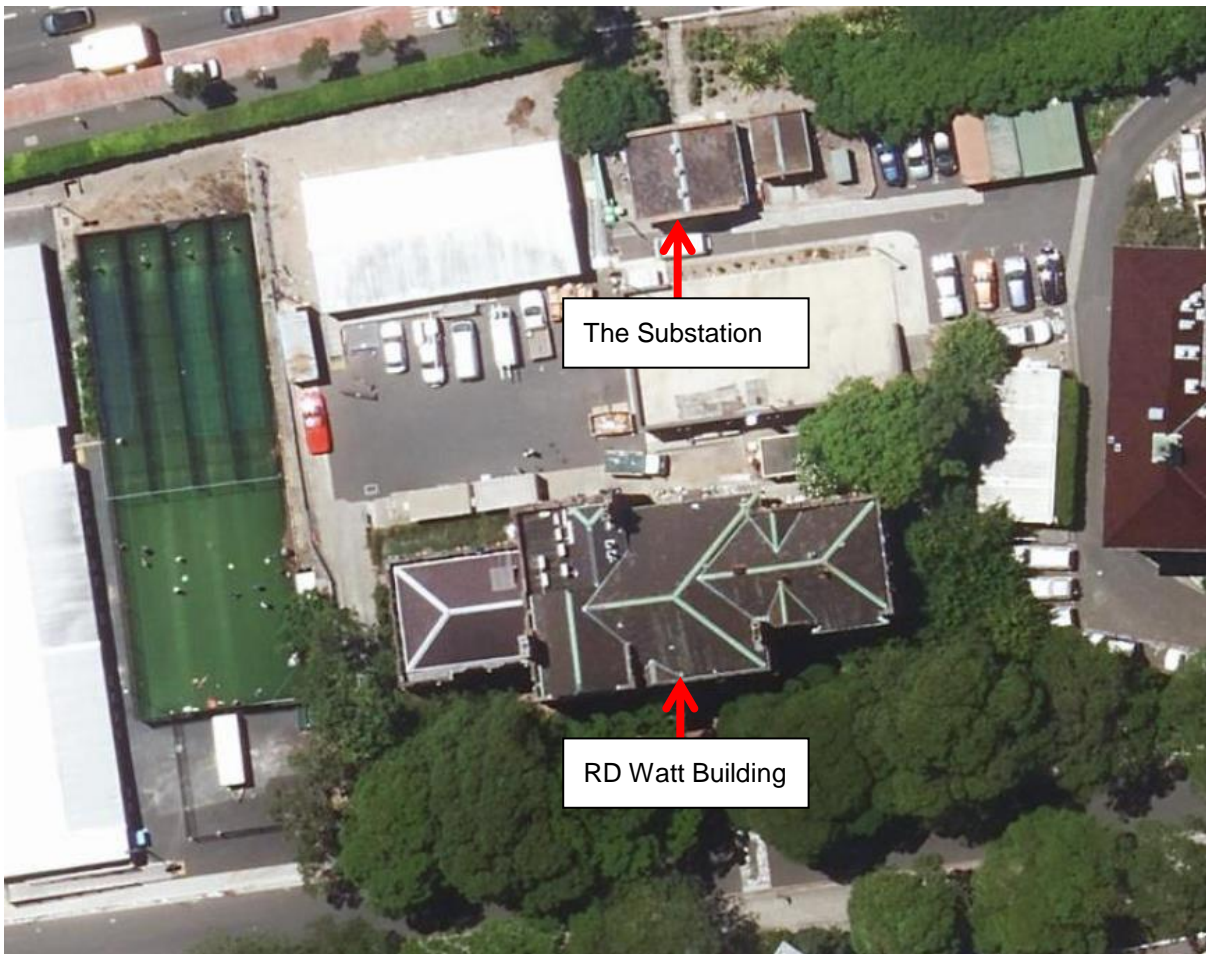
FIGURE 2 – AERIAL VIEW OF THE RD WATT BUILDING AND THE SUBSTATION
