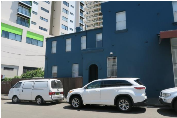
PICTURE 3 – VIEW OF THE SIDE (SOUTHERN) ELEVATION OF NO. 88 REGENT STREET
