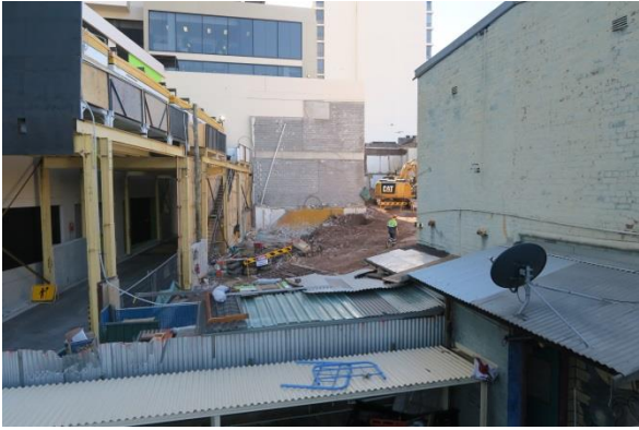
PICTURE 7 – VIEW OF NO. 60-78, SHOWING CONSTRUCTION WORKS IN PROGRESS
