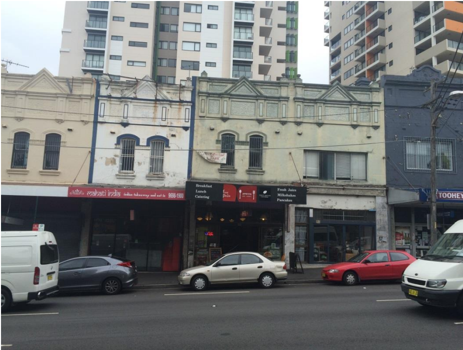
FIGURE 4 – EXTERNAL VIEW OF THE SUBJECT SITE FROM REGENT STREET, FACING WEST
