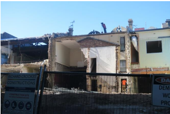
PICTURE 9 – VIEW OF NO. 60-78, SHOWING PARTIAL DEMOLITION OF BUILDINGS IN PROGRESS
