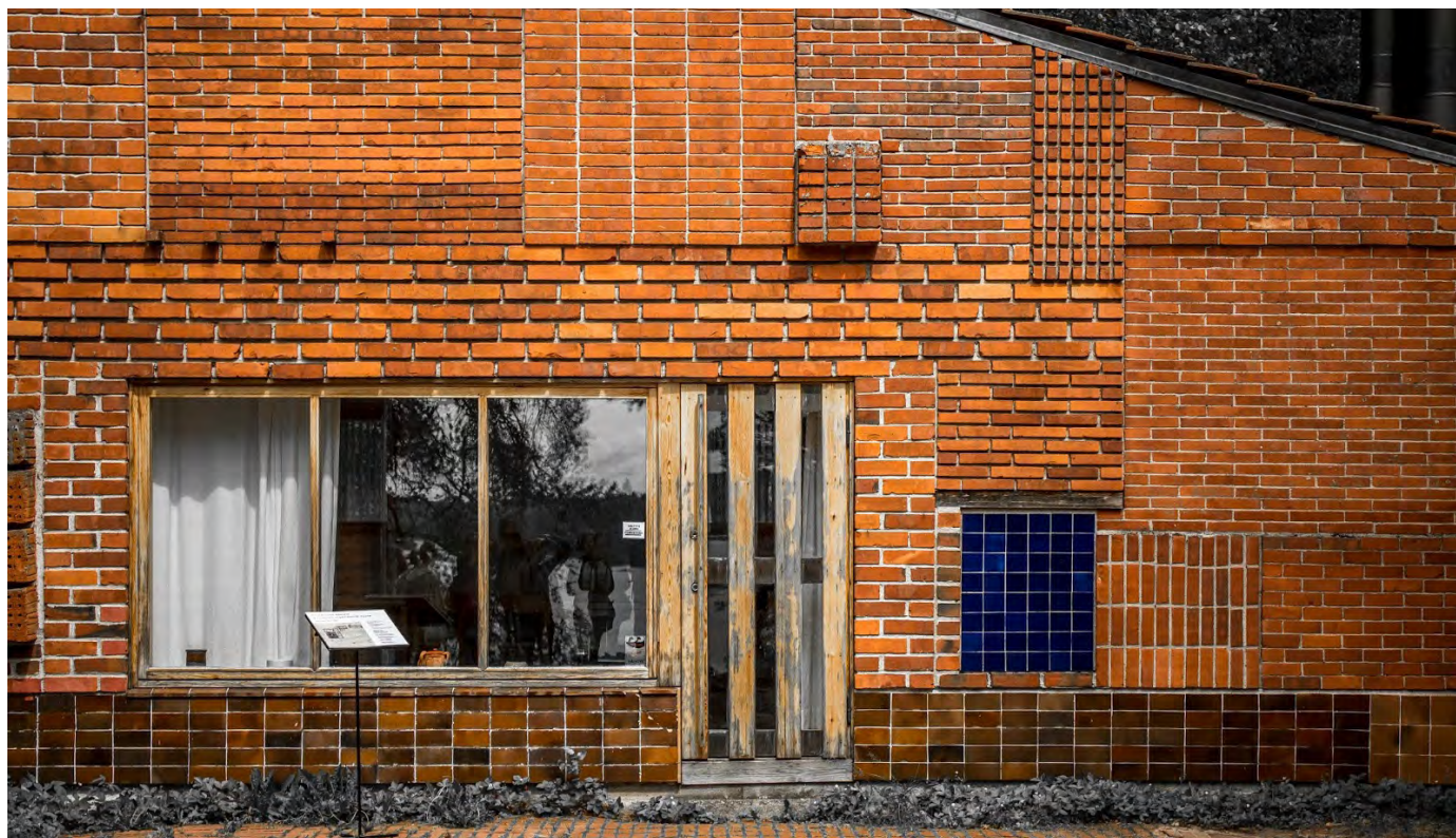
'Muuratsalo Experimental House' in Finland by Alvar Alto
