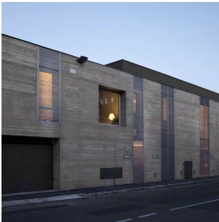
'Prato Lofts' in Prato, Italy by MDU Architects
