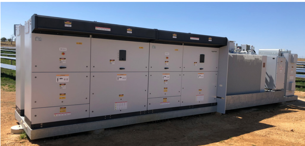
Photograph 3.2 Containerised inverter solution
