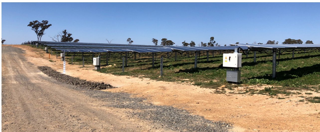
Photograph 3.1 PV module rows with single axis tracking technology
