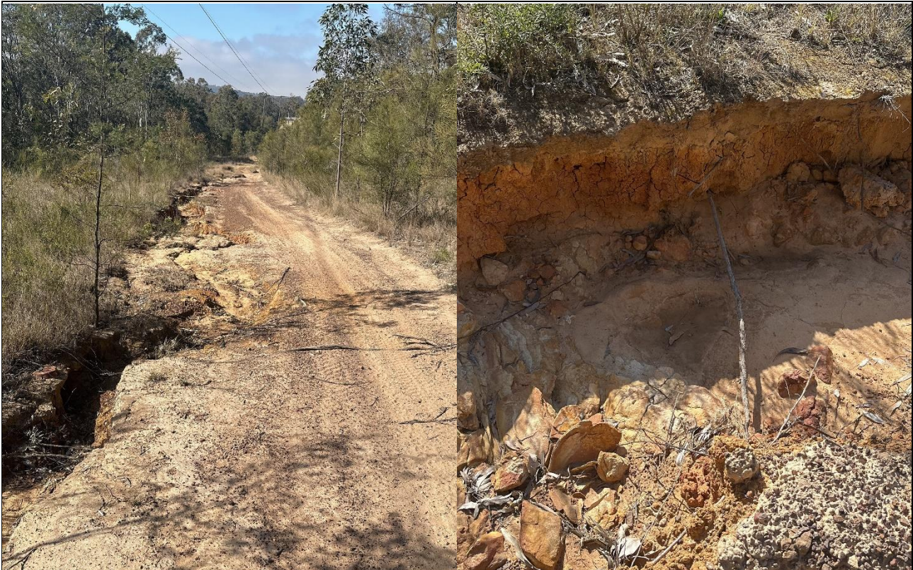
S09: SSA northern site boundary - significant rutting within easement access track (looking east)
