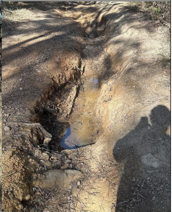
N10: NSA – significant rutting within access track adjacent rail line (looking southeast)
