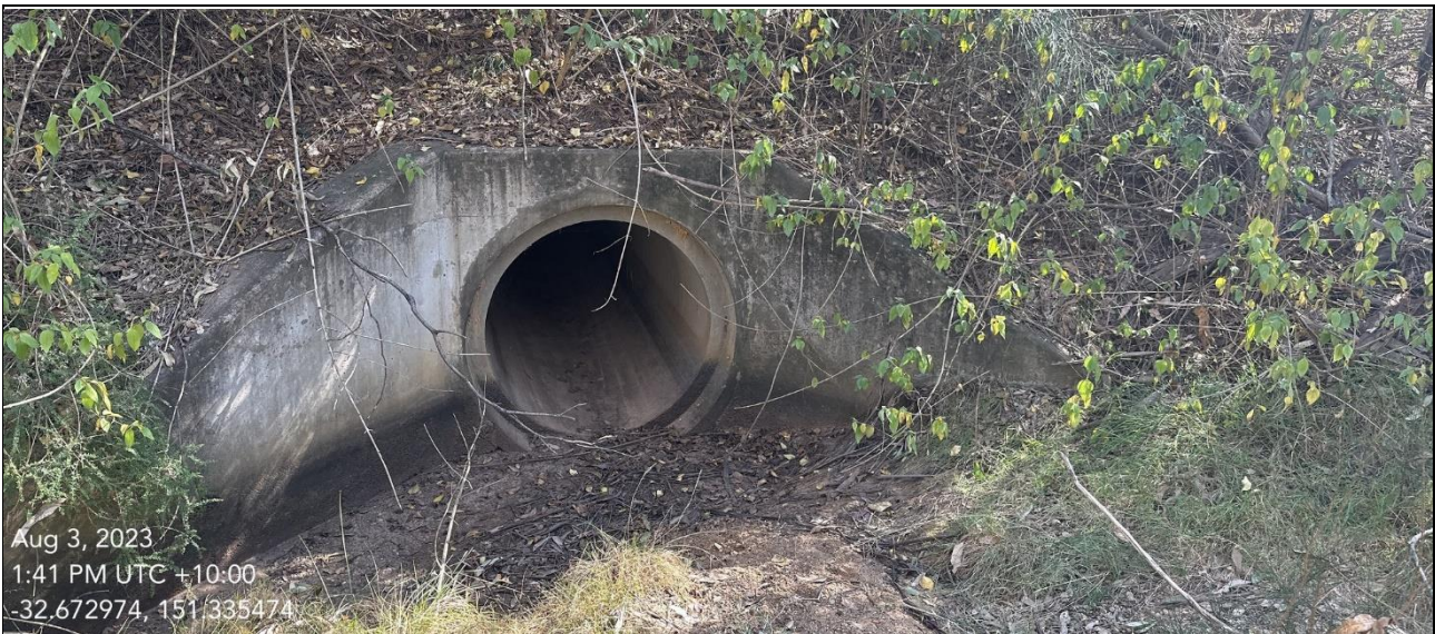
N11: NSA – existing concrete culvert inlet below approx. 5m high rail embankment (looking west)
