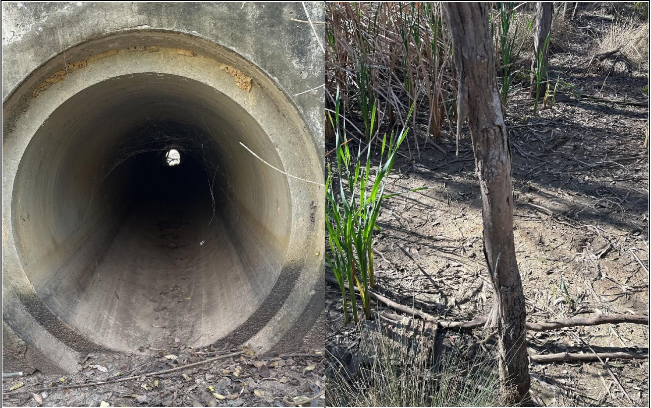
N12: NSA – existing concrete culvert (inlet side), no signs of significant blockage evident.
