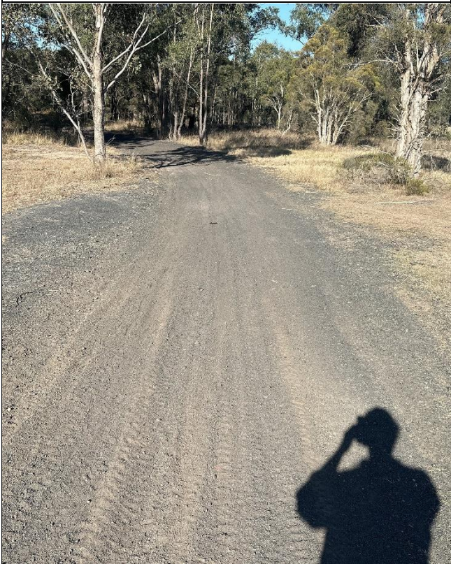
N22: NSA – chitter surfaced access track, southwest of site (looking east)
