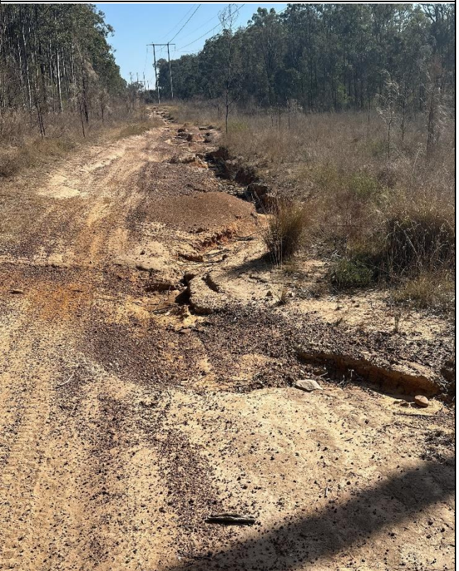
S08: SSA northern site boundary - significant rutting within easement access track (looking west)
