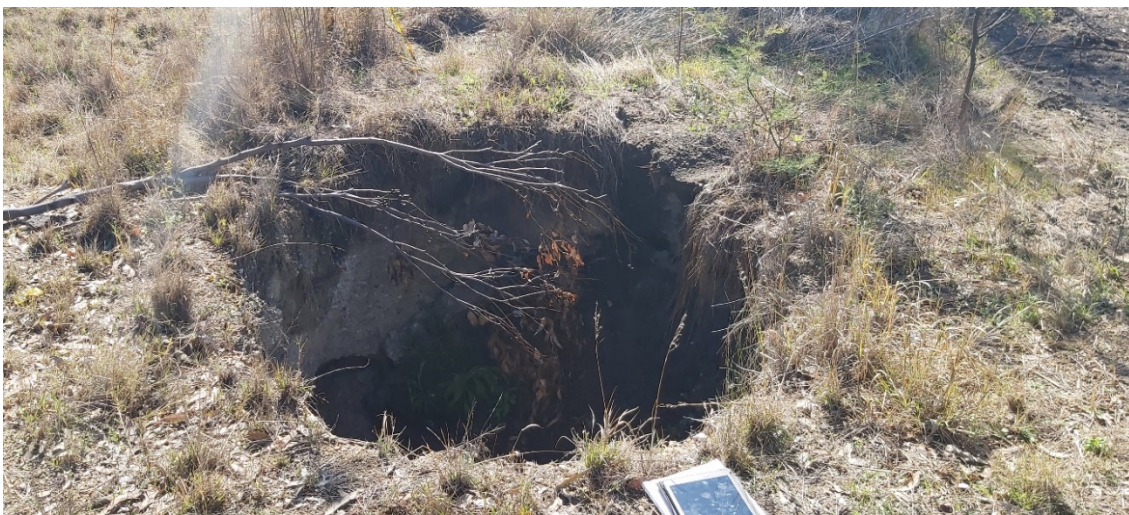
Photograph 2 Pothole – Stage 2 north (Village 3 Area)
