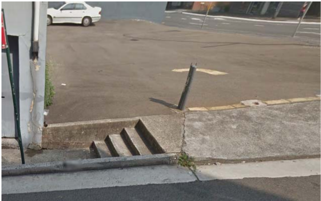
Figure 2: Stair located in the Woodburn Street footway
