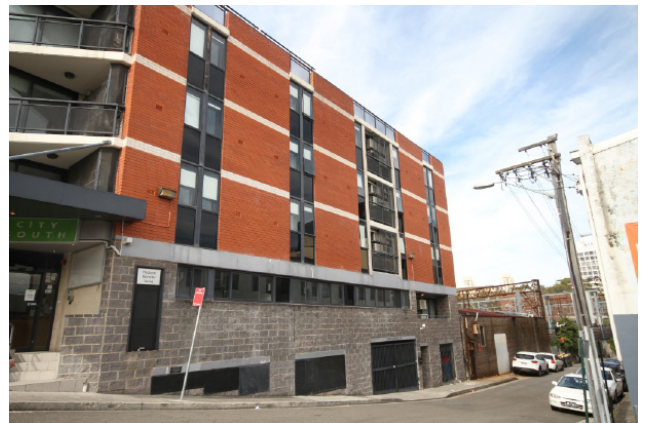
Figure 2.7 Corner of Cleveland and Woodburn Streets, showing the hotel adjacent to the subject site
