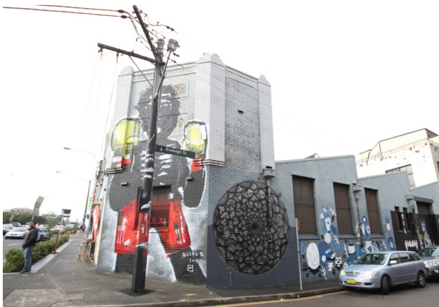
Figure 2.12 View of the splayed corner of the subject site on Cleveland and Eveleigh Streets, showing the two storeyed building stepping down to one storey at the rear.
