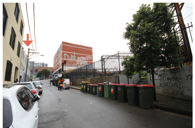
Figure 2.9 Woodburn Street view, looking towards Cleveland Street. 1-5 Woodburn Street is marked with a red arrow, and is adjacent to a 3 storey building.
