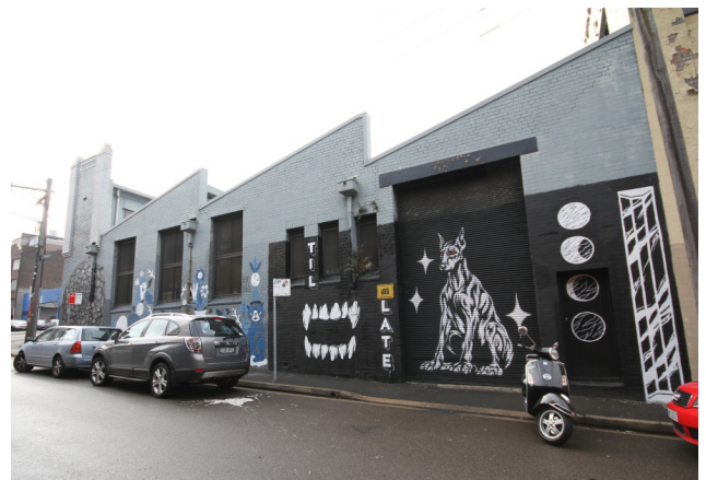
Figure 2.13 Eveleigh Street view of the subject building at 175 Cleveland Street, with its single storey form and saw tooth roof
