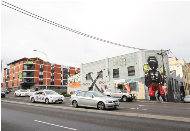
Figure 2.10 Main elevation of 175 Cleveland Street, with its splayed corner at Eveleigh Street
