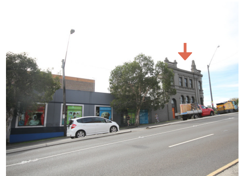
Figure 3.3 View across Cleveland Street, looking towards the listed heritage item at 151 Regent Street (marked with an arrow)
