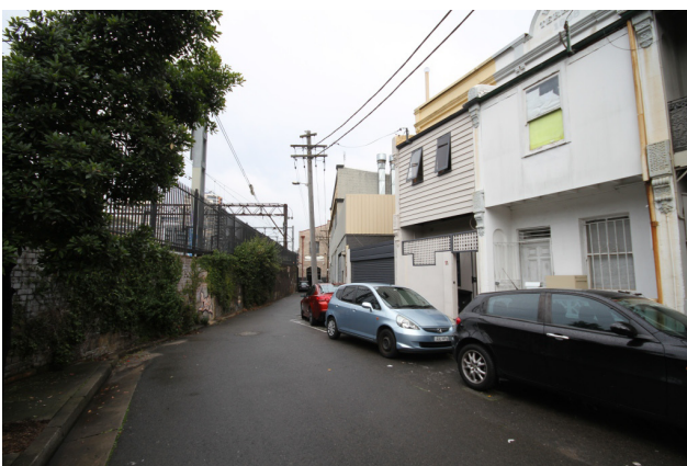
Figure 2.8 View looking along Woodburn Street, showing modified terrace houses in the vicinity of the site
