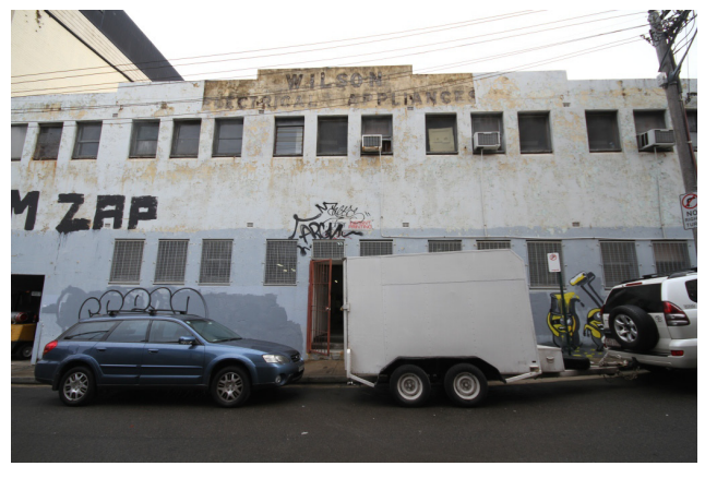
Figure 2.15 Main elevation of 1-5 Woodburn Street, showing its basic two storeyed form
