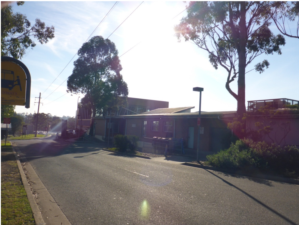
Plate 4 View north east overlooking the existing regional renal dialysis building and vehicle access way. RPS 2014
