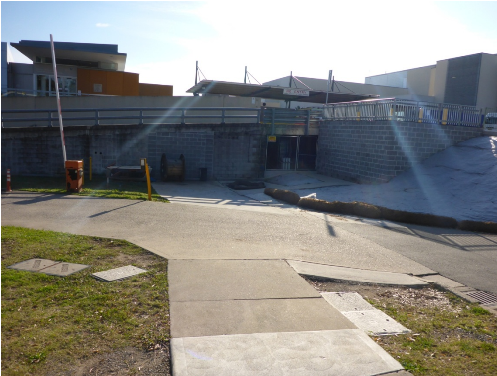
Plate 5 View of the benching for the new main entrance vehicle access ramp. RPS 2014
