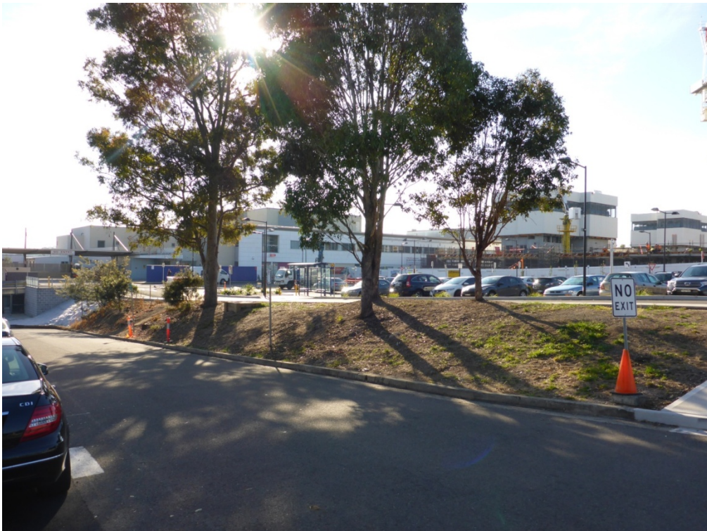
Plate 2 View north east overlooking an access road and car park showing evidence of landform modification and sub-surface services. RPS 2014
