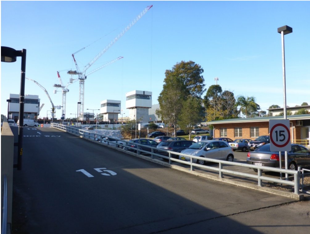
Plate 3 View south east overlooking the new vehicle access ramp with the existing regional renal dialysis buildings to the right of the plate. RPS 2014
