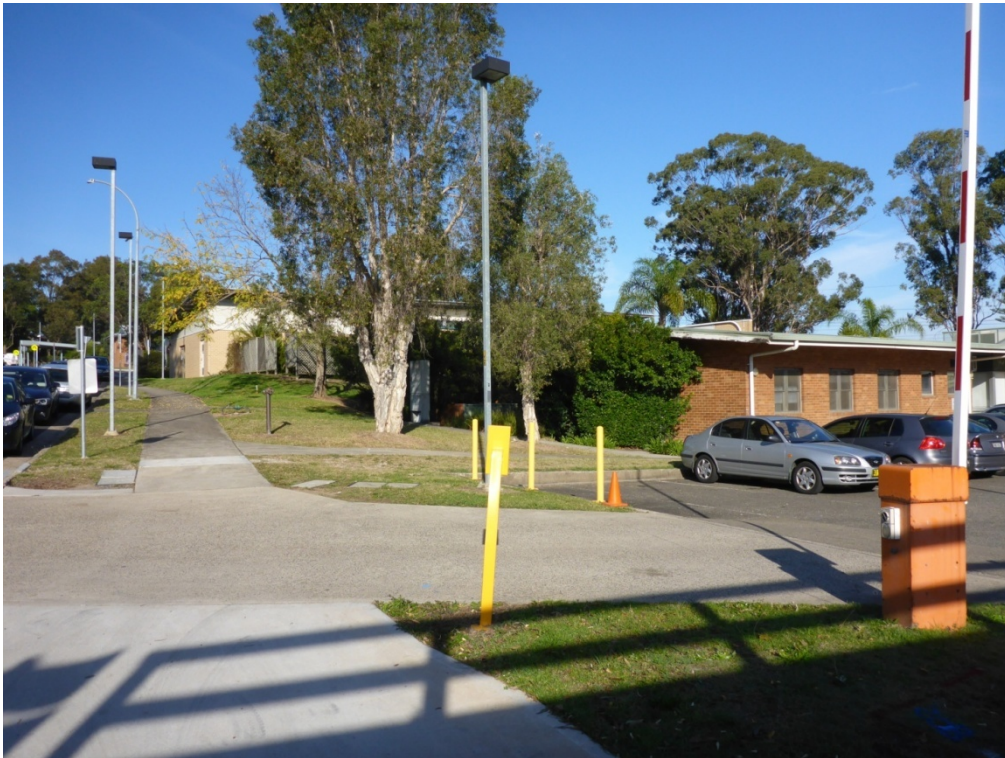
Plate 6 View south west overlooking the existing regional renal dialysis buildings and associated infrastructure, services and landform modification. RPS 2014
