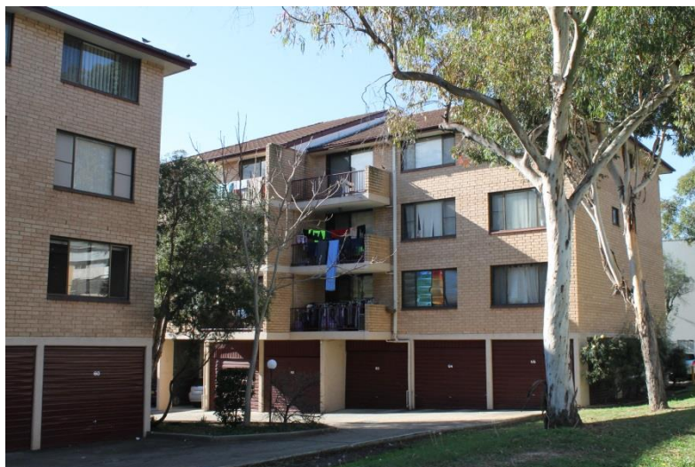
Figure 15 – Residential Development on the northern side of Blacktown Road Source: JBA
