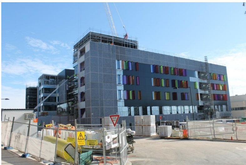
Figure 5 – New 6 storey CSB building Source: JBA
