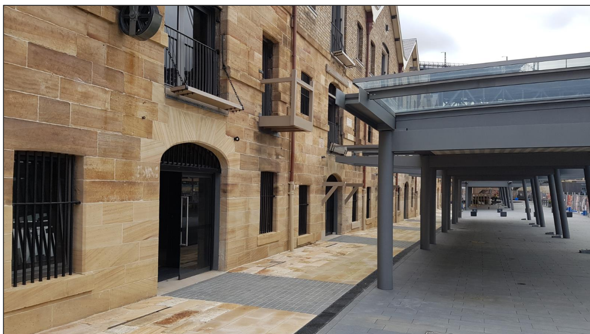
Figure 4 Photo of the eastern façade along the harbour foreshore (Source: Photo taken 3 April 2019)
