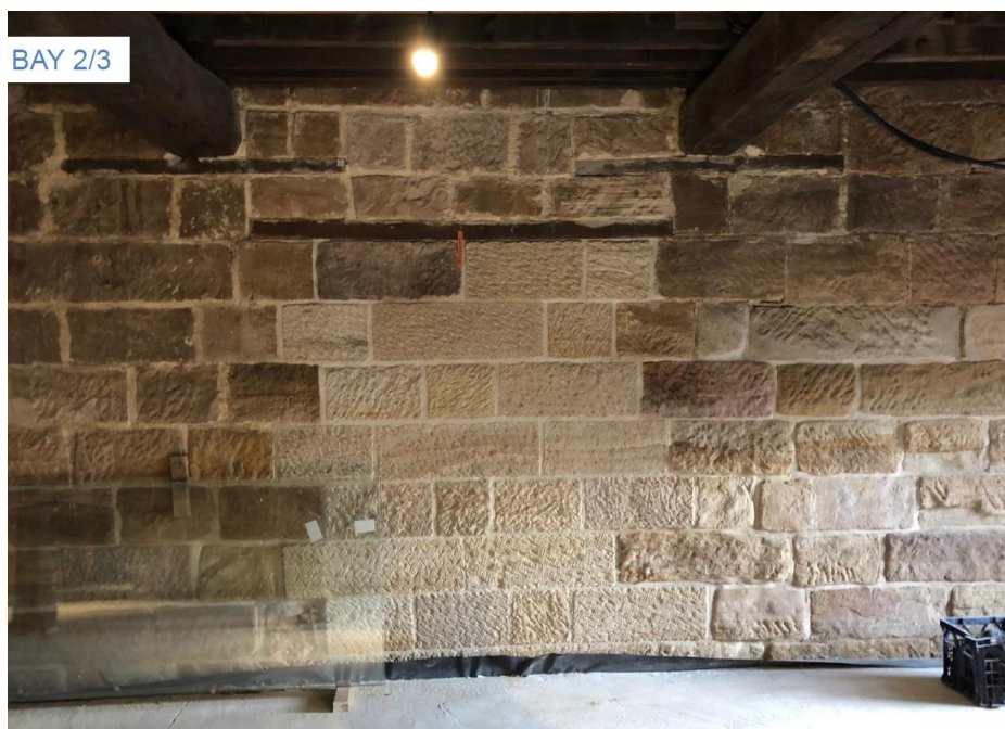
Figure 4 – Photo of Ground Level Bay 2 / 3 showing new fabric to be removed
