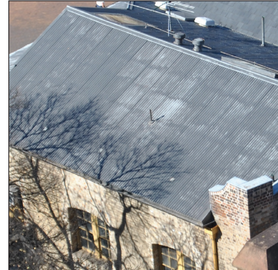
MS Metal roof sheet to match existing
