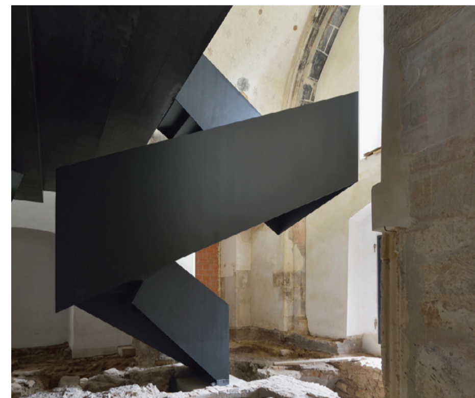
Steel fabricated stair finished with warm grey tone MIO paint
