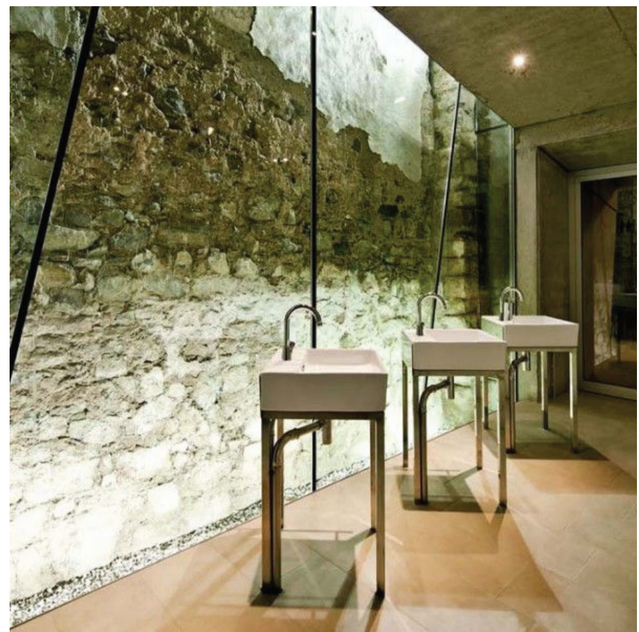
GL1 Low iron glass, Frameless glazing, clear glass, non-reflective and with neutral (not tinted, green or grey) body tint.
