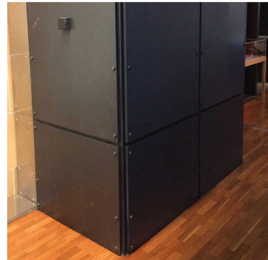
MP1 Express jointed metal bonded marine grade plywood/ cfc panels finished with MIO paint
