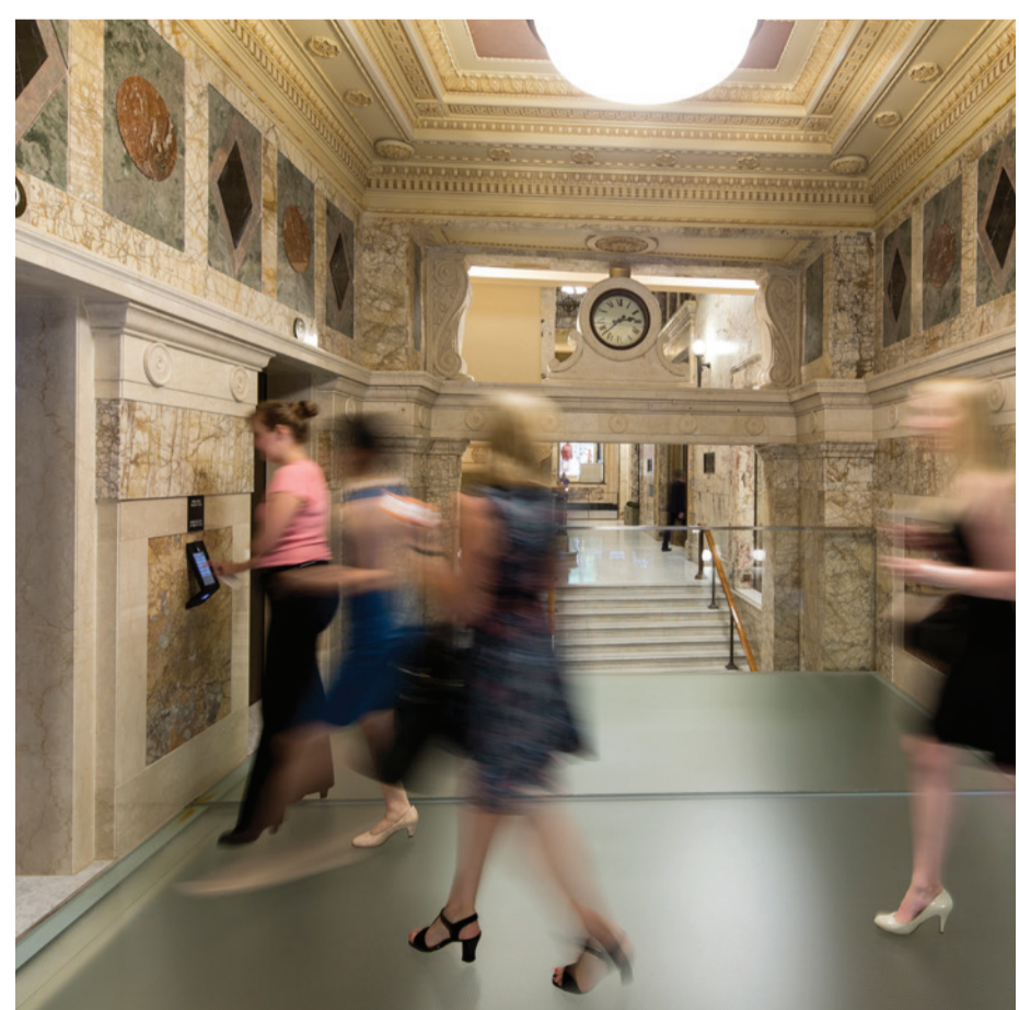
GL3 Acid etched slip resistant Glass floor; obscure treatment to match 50 Martin Place project Benchmark.
