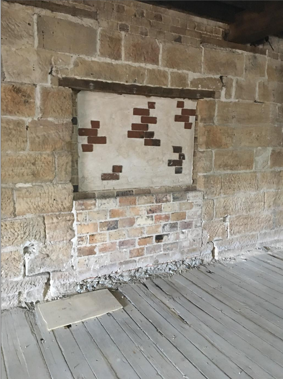
Figure 6 – Picture of bricked up opening at Bay 8–9
