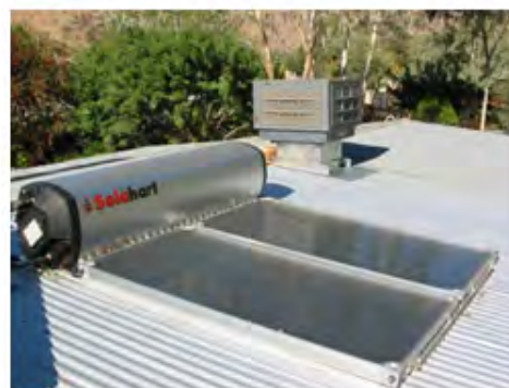
Figure 12 Solar hot water system
