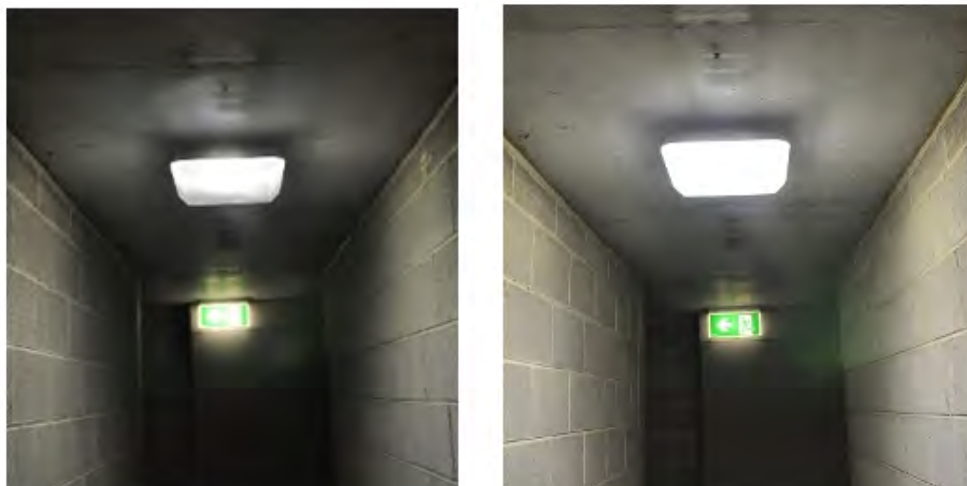
Figure 9 Emergency lights in standby & occupancy modes
