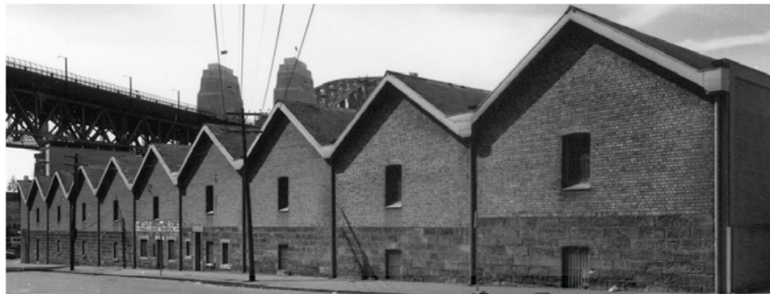
Figure 1.2 Photograph from 1970 showing original windows, later modified to
