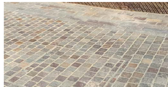
Figure 2.2 Photograph from Barangaroo Headland Park, indicating a granite-set paver complying with wheelchair accessibility, and consistent with the proposed specification (Figure 2.3, right).
