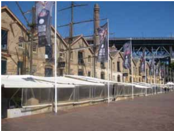
PICTURE 1 – OUTDOOR DINING AREA ALONG FORESHORE PROMENADE
