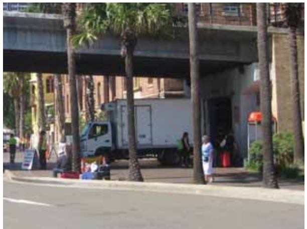
PICTURE 6 –LOADING DOCK IN CIRCULAR QUAY WEST
