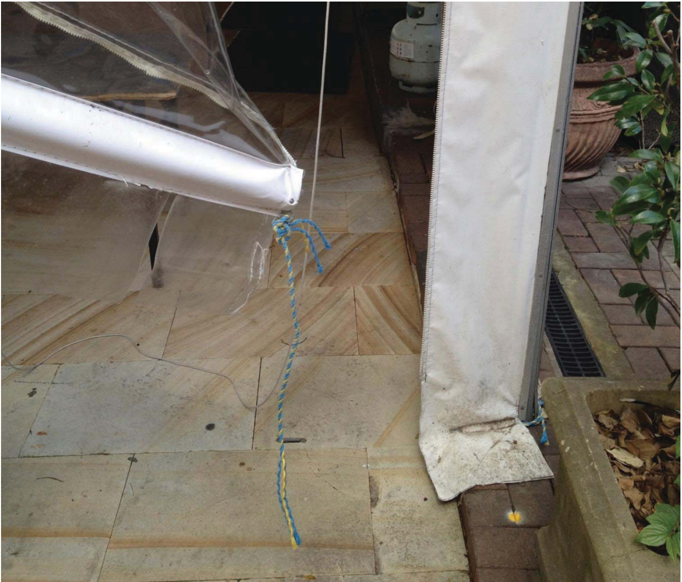
Figure 6: The existing ground covering is Sandstone paving. This paving appears to be in good condition suggesting that it is possible that minimal significant tree roots will be found directly beneath this surface.
