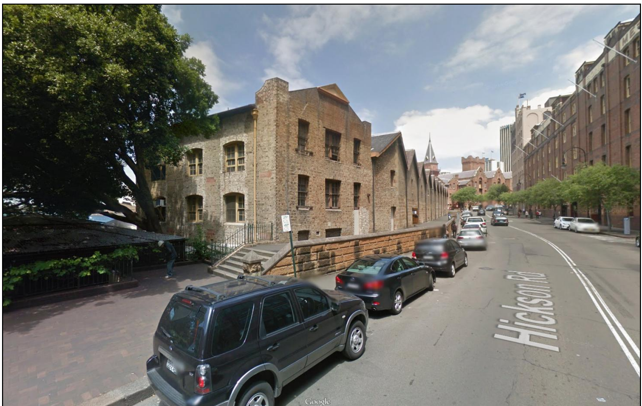
Photo 2: View of existing Campbell's Stores, looking south from Hickson Road
