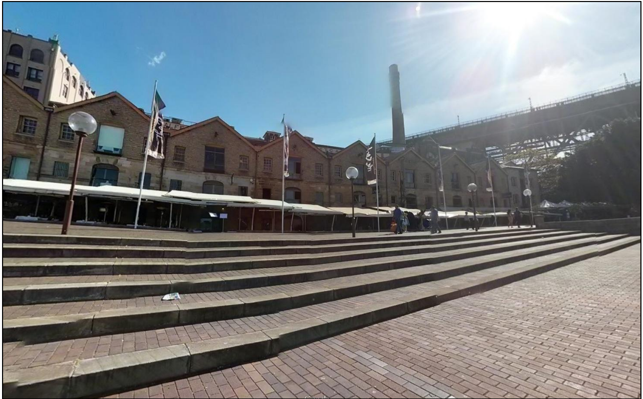
Photo 5: View of existing Campbell's stores, looking north-west from the eastern frontage of the site
