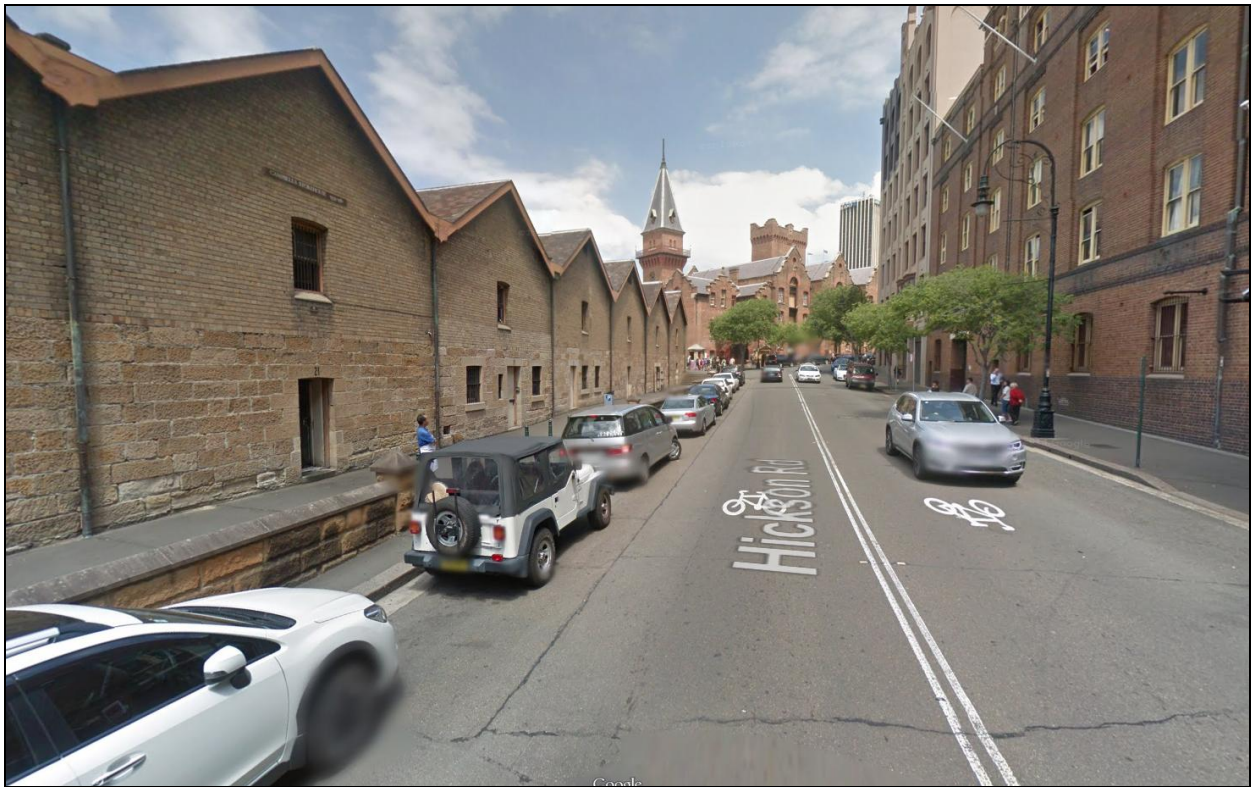
Photo 3: View of existing Campbell's stores, looking south from Hickson Road
